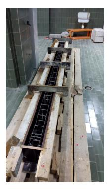
FIGURE 3.14: Reinforcement in the formwork
