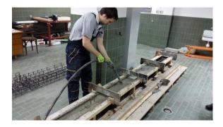
FIGURE 3.16: Placing concrete in the formwork
