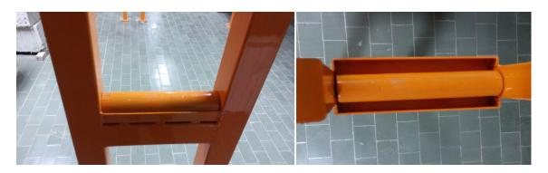
FIGURE 3.28: Steel support roller – fixed (left) and free (right)
