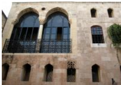
Figure 4.12: Ashlar and dressed quarry stone walls used in the old houses in Damascus.
