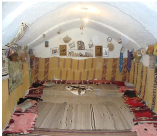
Figure 8.42: Roof is in the form of a barrel vault.
