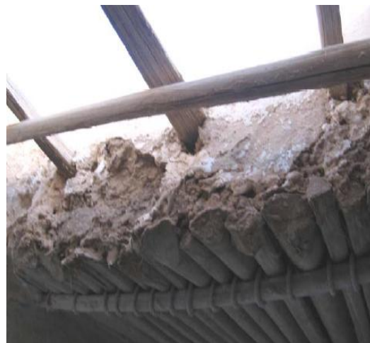
Figure 8.63: The ceiling consists of stumps from the palms, and small stones and stones.
