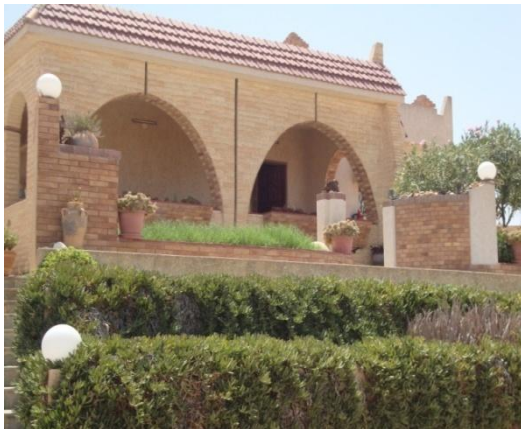
Figure 8.45: North façade of Arabi Belhadj house in Gharyan.
