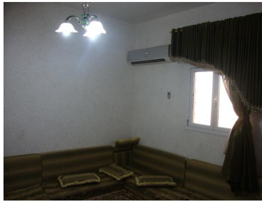
Figure 8.71: Bedroom equipped with air-conditioning in Hussein Mohamed house in Ghadames.
