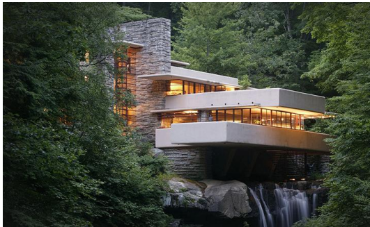
Figure 2.1: The way the block-like house is constructed out of a waterfall is inspirational. ( http://en.wikipedia.org/wiki/Fallingwater ) (January 2015).
