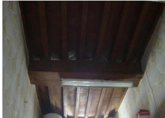
Figure 8.2: Timber ceiling in Mahmoud Sola house in Tripoli.
