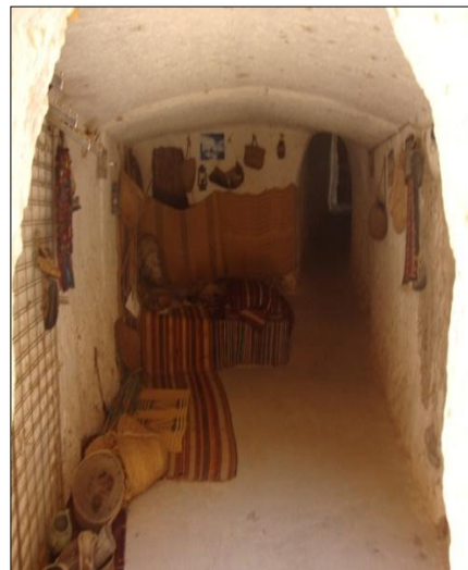
Figure 8.35: The ceiling of the corridor is equal to a half of the arch.
