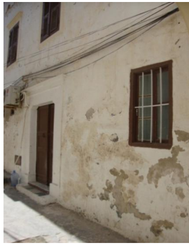
Figure 8.5: Façade painted by white color of Mahmoud Sola house in Tripoli.
