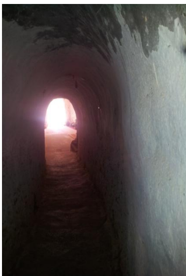
Figure 8.35: The ceiling of the corridor is equal to a half of the arch.
