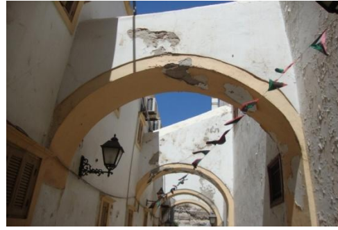
Figure 6.2: Arches are built between one house and another all along the street.
