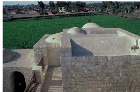
Figure 2.4: Roof view. ( http://archnet.org/ ) (February 2015).
