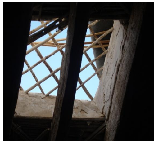
Figure 8.65: Opening at the roof.
