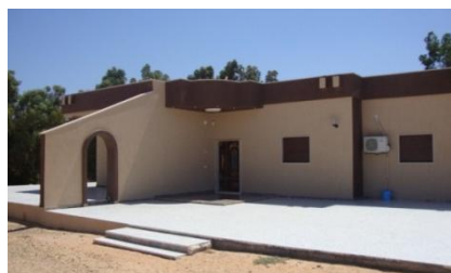
Figure 8.19: Air-conditioning system of Abdalmast Shahrani house in Tripoli.
