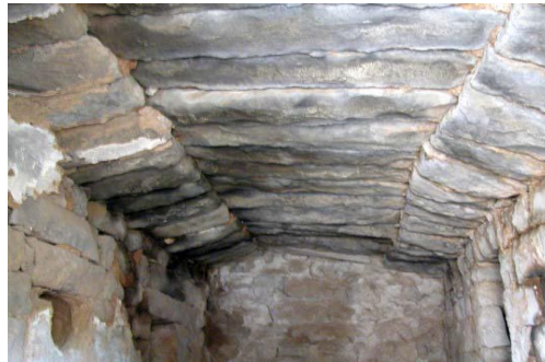
Figure 4.13: A stone roof used in the southern areas of Syria.
