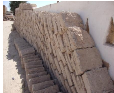
Figure 8.55: Bricks made of clay and dried in the sun, with dimensions 10cm x 30cm x 40cm.
