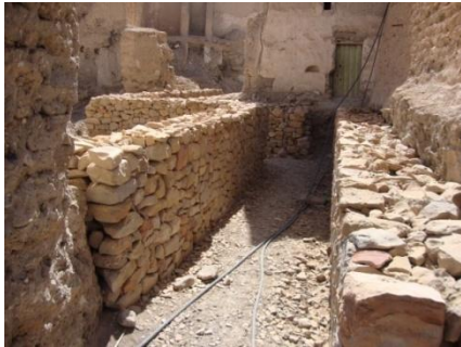
Figure 8.54: Granite stone is used for the foundations.
