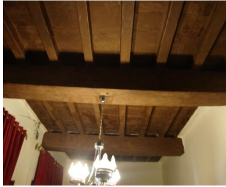
Figure 6.10: Roof of a room.
