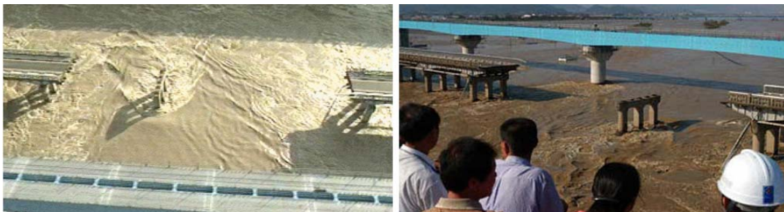
Fig. 1.2 Gupo bridge on the Nakdong river, South Korea, 2003, [Ji and Julien 2005]
