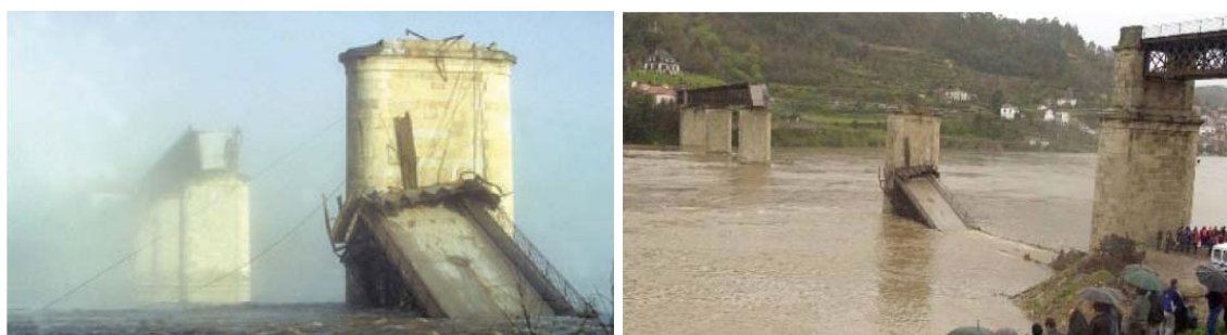
Fig. 1.9 Collapse of the Hintze Ribeiro bridge, Portugal, 2001, [Figueiredo et al., 2013]
