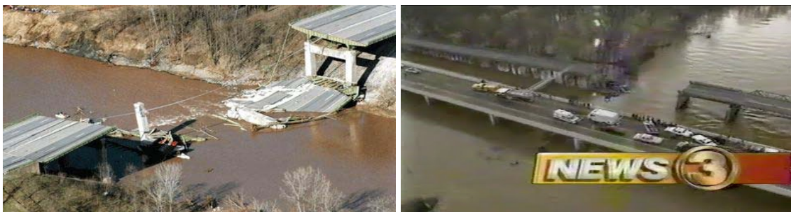
Fig. 1.5 The collapses of the Schoharie Creek Bridge, 1987 (left) and Hatchie River Bridge, 1989 (right), USA
