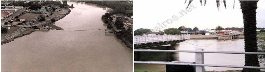
Fig. 1.8 Wairoa Bridge failure, New Zealand, 1988, [Wairoa, n.d.]
