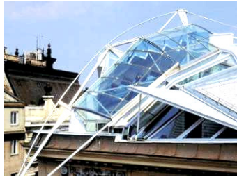
Rooftop Remodeling, 1983-88 Vienna
