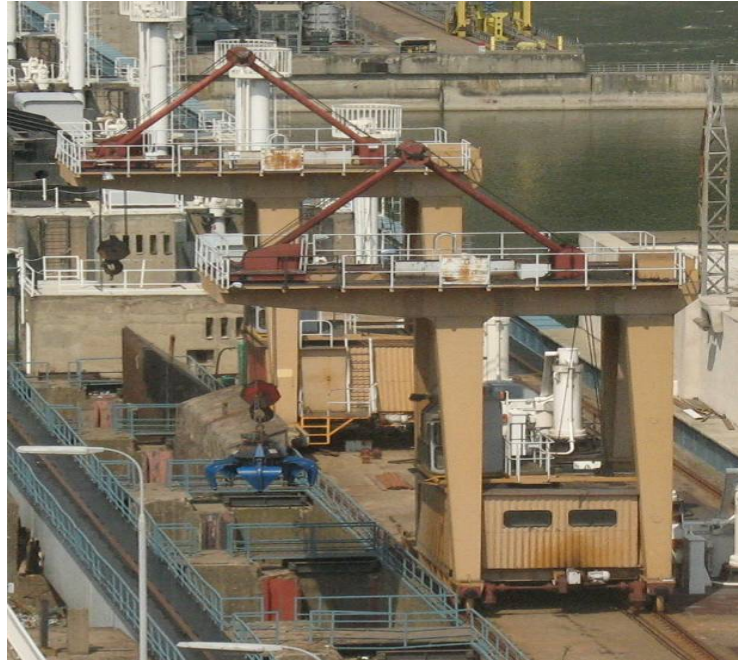
Figure 6.5: Gantry cranes in- situ, Model 2.
