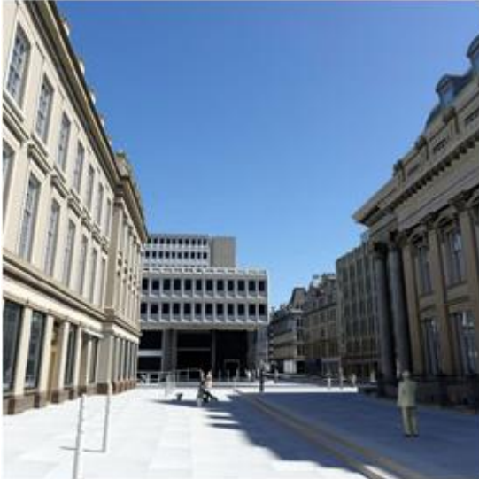
110 Queen Street as existing
