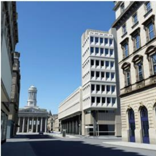
110 Queen Street as existing
