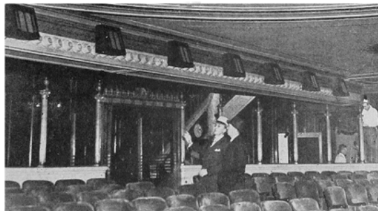
FANTASOUND INSTALLATION. Upper left, amplifiers and independent soundhead; 3-banks of speakers behind screen (upper right); additional speaker units are located in the auditorium (lower left and center). Simplex Projectors project the picture (lower right).
