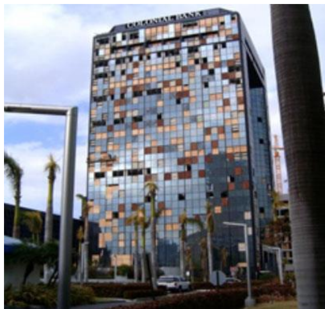
Slika 4.11. Oštećenja fasade tokom uragana Wilma, Miami 2005 (Beers 2011) https://buildingenvelope.files.wordpress.com/2011/05/wilma.jpg
