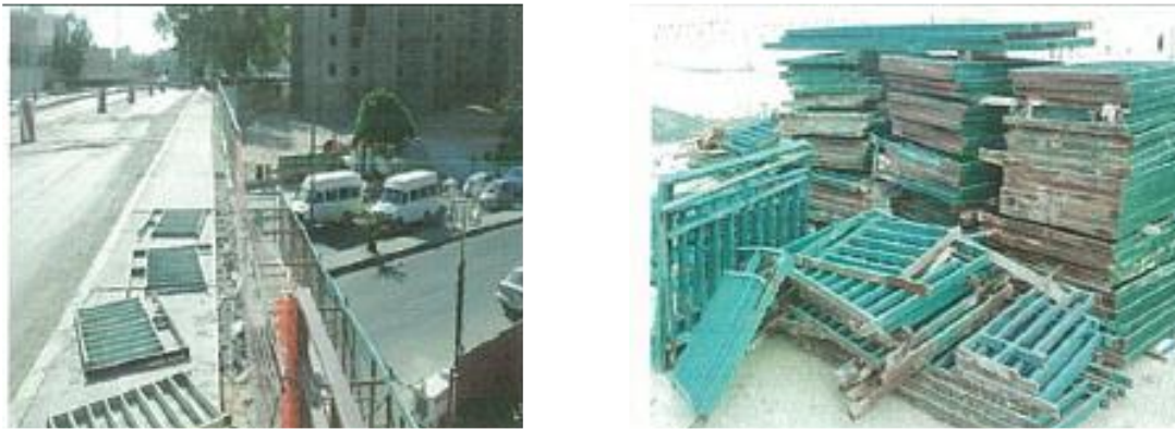
Figure (VIII-89). Removal of old fence
