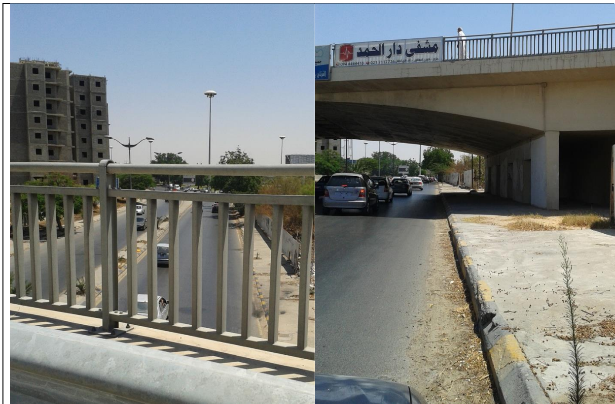
Figure (IX-61) A general view of fences on the bridge
