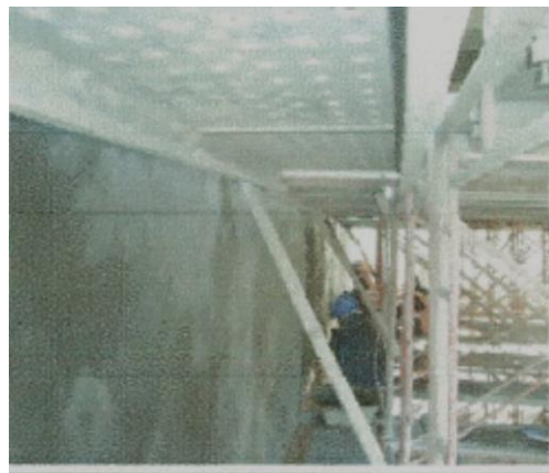
Figure (VIII-147) Execution of new cover on ceiling of bridge superstructure by plastering
