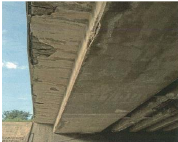
Figure VI-146. Cantilever slabs with damaged concrete (south side): delamination of concrete due to corrosion of rebars and running down of water
