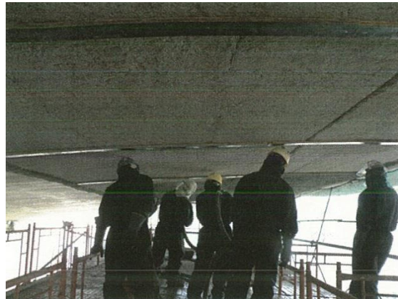
Figure (VIII-77) Preparing for plastering ceiling
