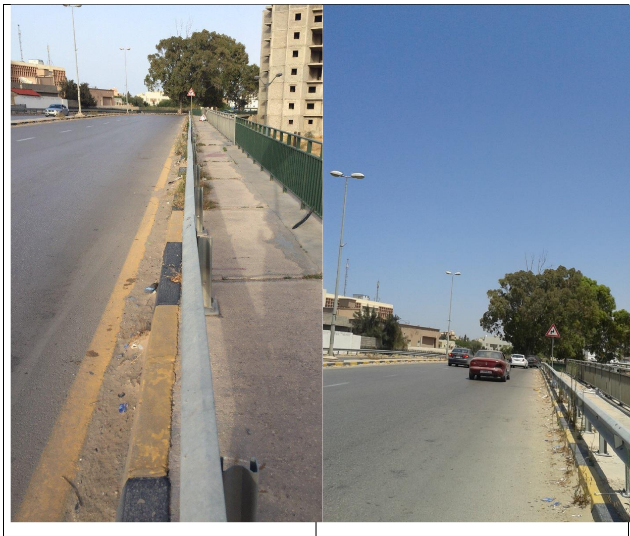
Figure (IX-59) A general view of asphalt wearing layer
