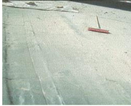
Figure (VIII-91). The view of surface after asphalt was removed
