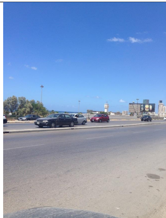
Figure (IX-16) A general view of Asphalt wearing layer
