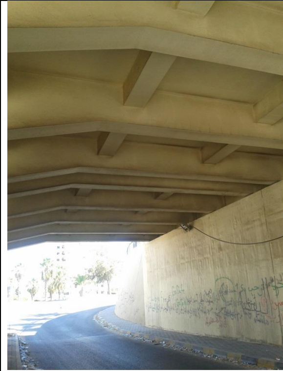
Figure (IX-140) A general view of main and secondary beams of superstructure of bridge
