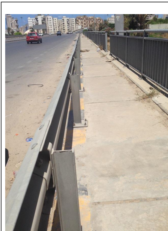
Figure (IX-15) A general view of Pedestrian path on bridge
