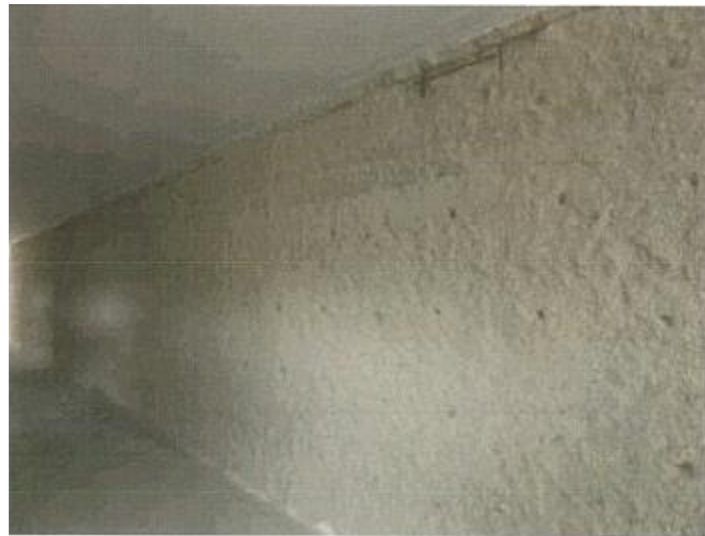
Figure (VIII-72) Damaged concrete cover removal from interior walls
