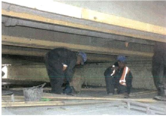
Figure (VIII-146) Reprofiling of lateral slab beams, bottom part
