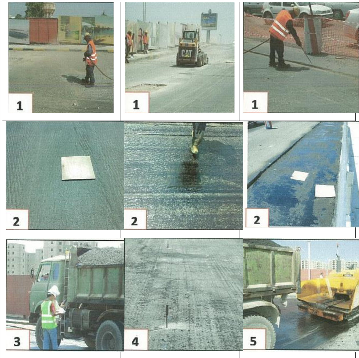
Figure (VIII-94). Phases of placing of bituminous materials
