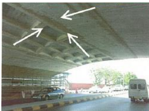
Figure (VIII-74) Local removal work on ceiling
