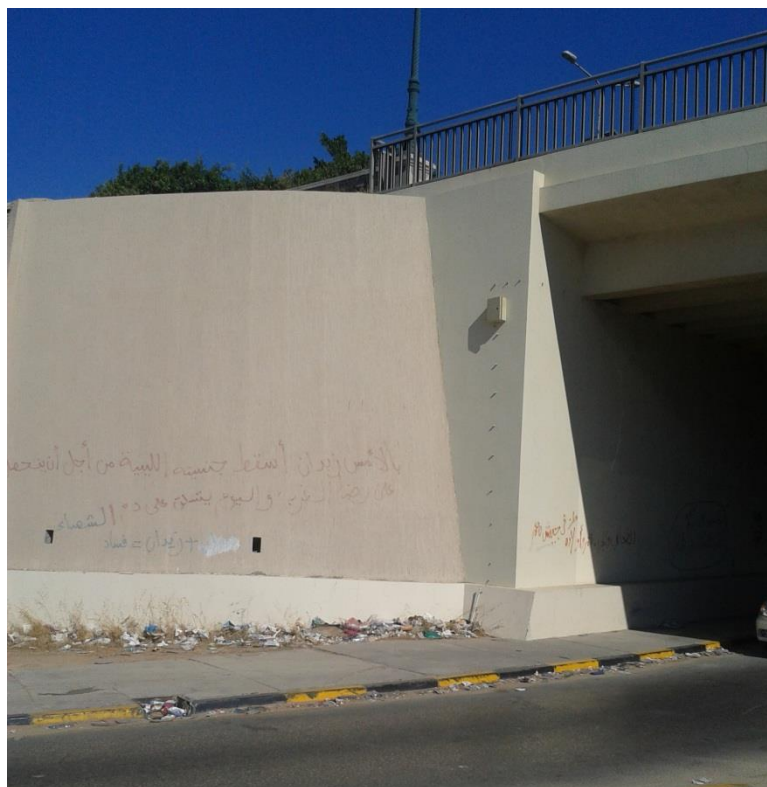
Figure (IX-129) A general view of catch pit under the bridge
