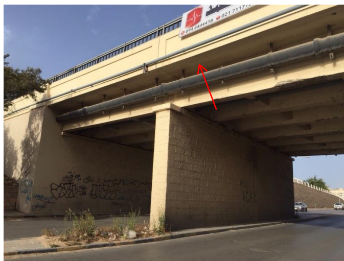
Figure (IX-97) View of cantilever slab
