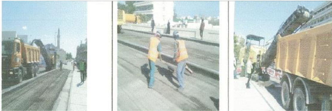
Figure (VIII-154) Removing existing asphalt wearing layer, reclaimed asphalt
