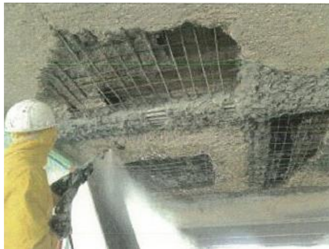
Figure (VIII-8): Rebars cleaning with water-sand blasting in deck ceiling slab
