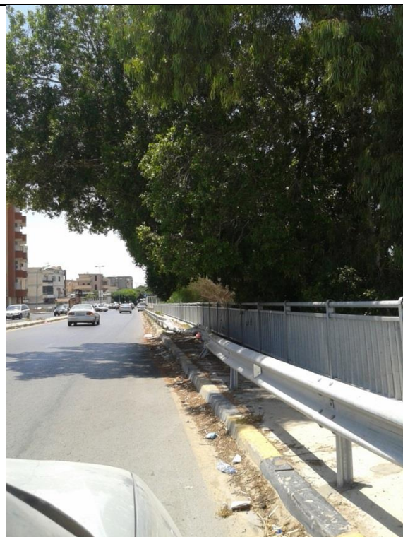
Figure (IX-88) A general view of curbs
