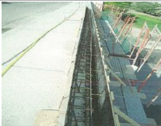
Figure (VIII-28) Reinforcement for new beam
