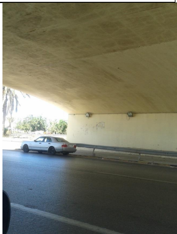
Figure (IX-34): Look of deck ceiling and abutments
