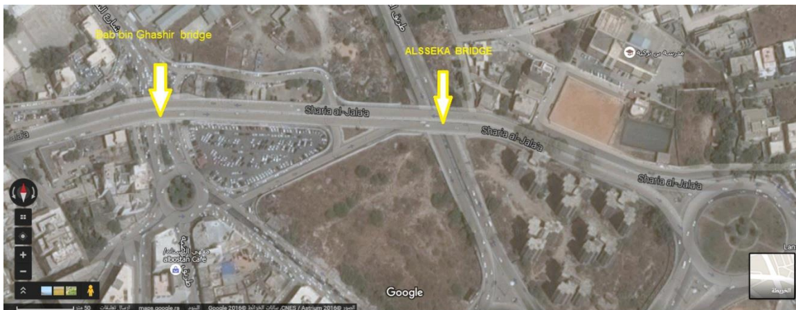
Figure VI-58. Alsseka Road Bridge location on Google Maps
