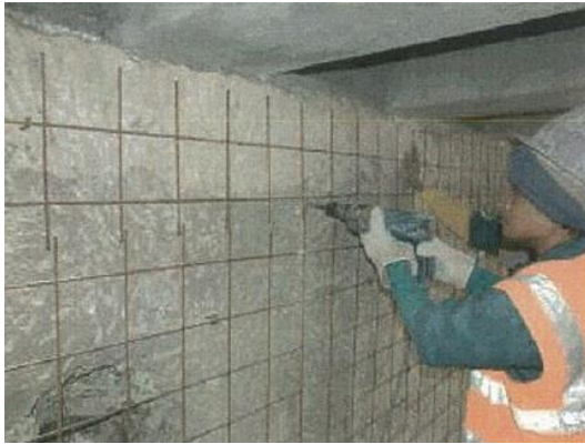
Figure (VIII-168) Abutment wall wire mesh application
