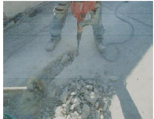
Figure (VIII-141) Damaged plastering and concrete removal from the abutments and sidewalk
