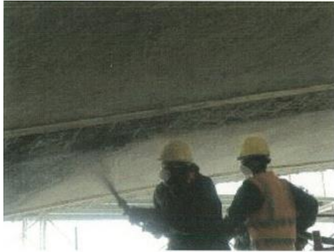
Figure (VIII-15) cementitious base special mortar on deck ceiling beams
