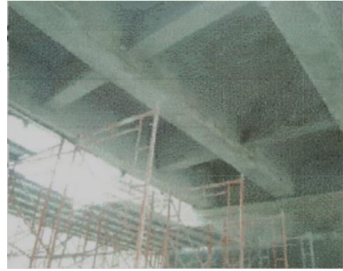
Figure (VIII-147) Execution of new cover on ceiling of bridge superstructure by plastering
