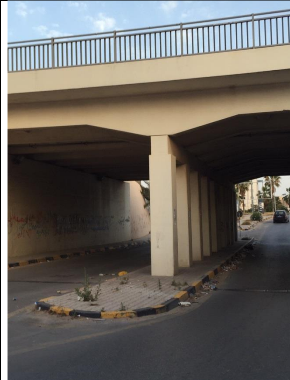
Figure (IX-132) A View of columns which were strengthened by enlarging cross sections
