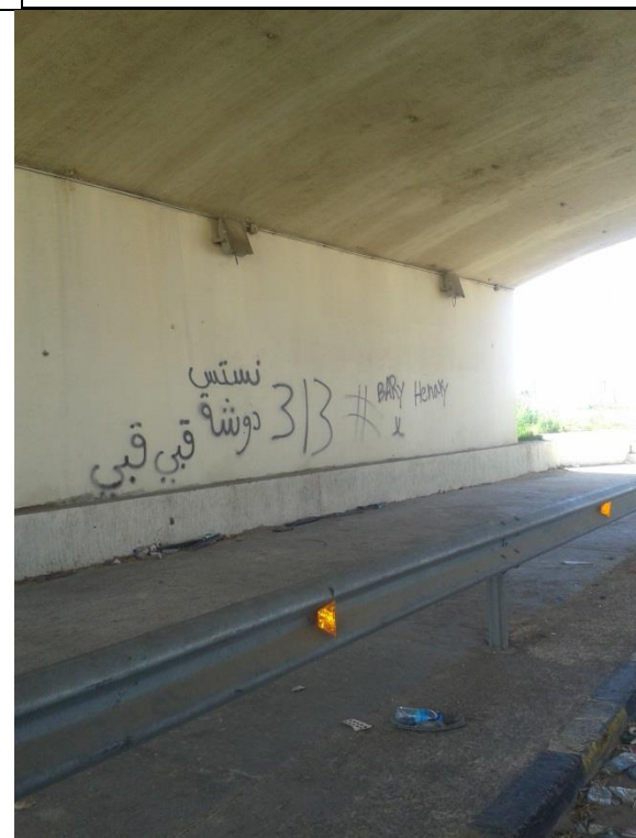
Figure (IX-33): View of supporting wall
