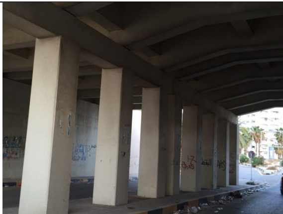
Figure (IX-134) A View of strengthened columns
