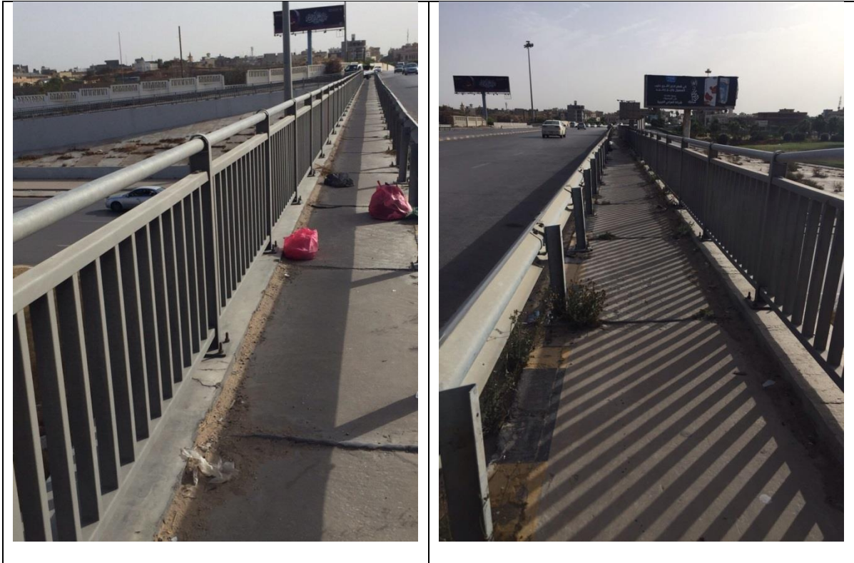
Figure (IX-35): View of pedestrian path
