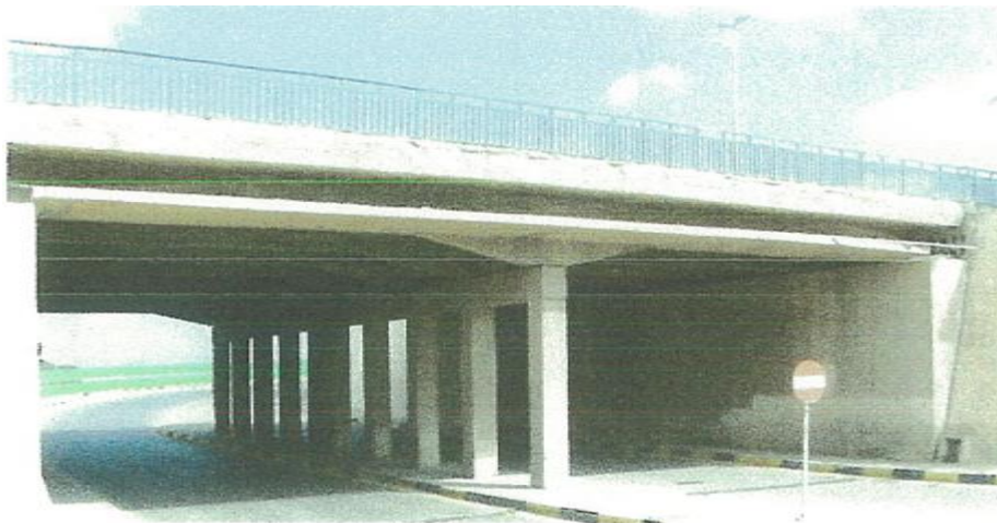
Figure VI-151. Abdul Salam Aref bridge aspect
