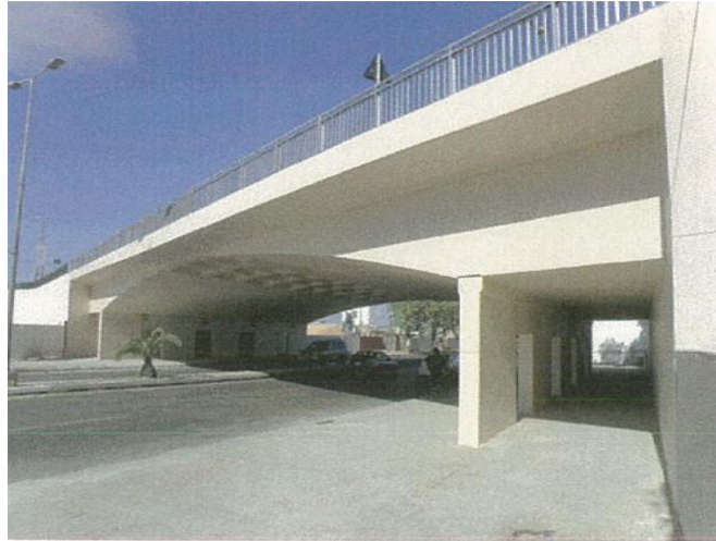
Figure VI-59. Alsseka bridge interior wall and arch cantilever
