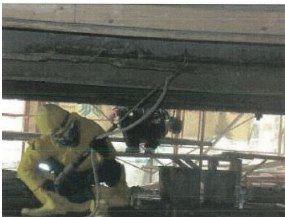
Figure (VIII-142) Cleaning of rebars with water-sand blasting, deck ceiling beams
