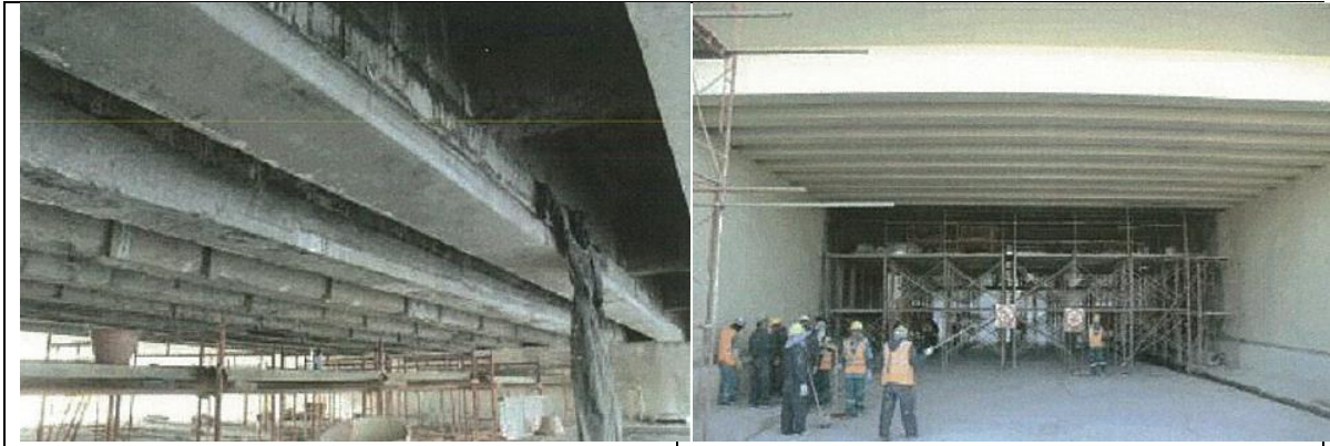
Figure (VIII-166) Longitudinal slab beam bottom repaired
