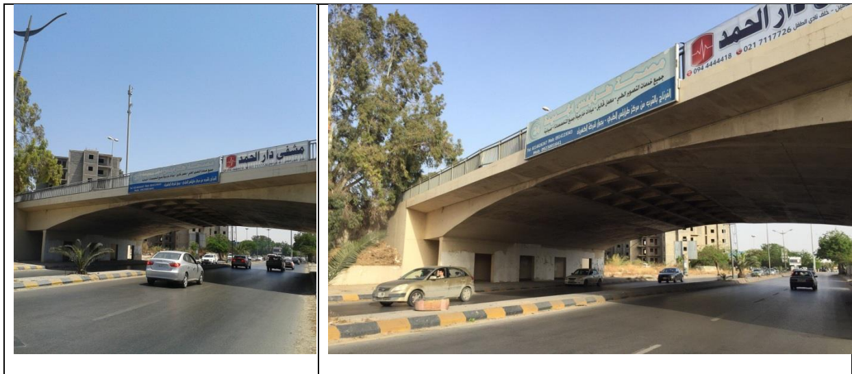
Figure (IX-43) A general view of Alsseka Road Bridge
