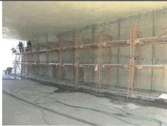
Figure (VIII-115) Abutment wall repair
