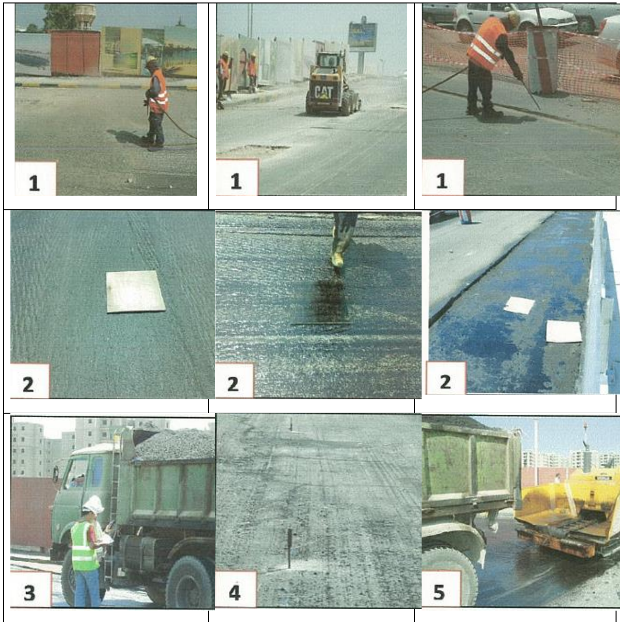
Figure (VIII-132) Phases of placing of bituminous materials
