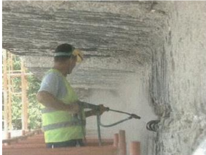
Figure (VIII-105) Rebars cleaning with water-sand blasting
