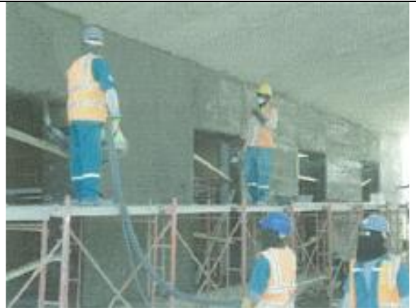
Figure (VIII-116) Plastering of supporting wall
