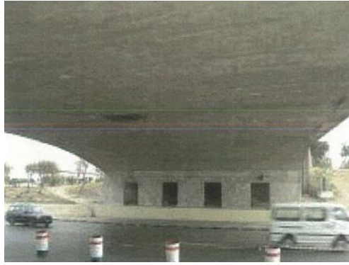
Figure VI-3. Souk Athulatha1 detail of ceiling and exterior wall
