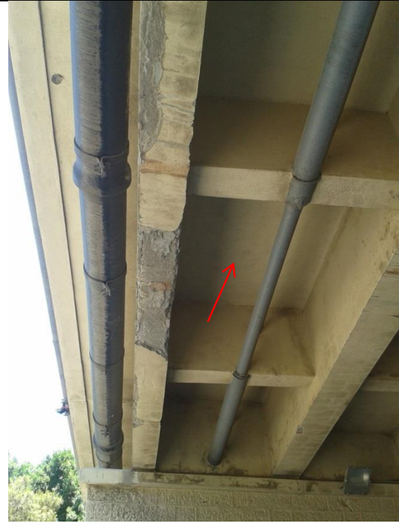
Figure (IX-93) View of deck slab, longitudinal and transversal supporting beams
