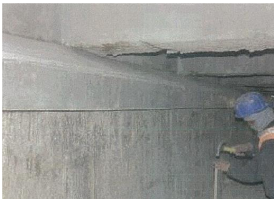
Figure (VIII-146) Reprofiling of lateral slab beams, bottom part
