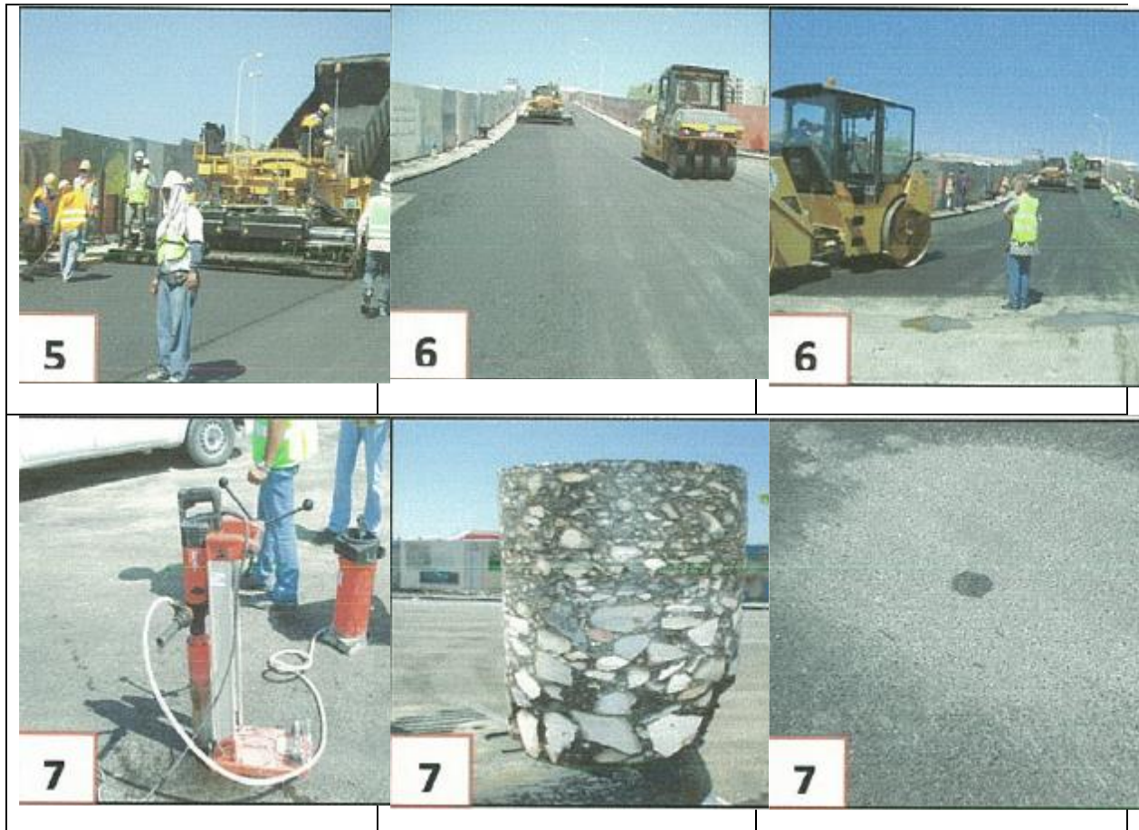
Conti. ....Figure (VIII-132) Phases of placing of bituminous materials
