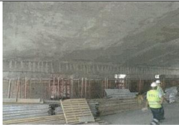
Figure (VIII-108) Finalizing underpass ceiling with special mortar
