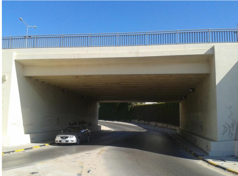
Figure (IX-109) A general view of Al shaab port bridge
