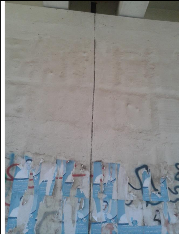
Figure (IX-138) Look of expansion joint between two abutments
