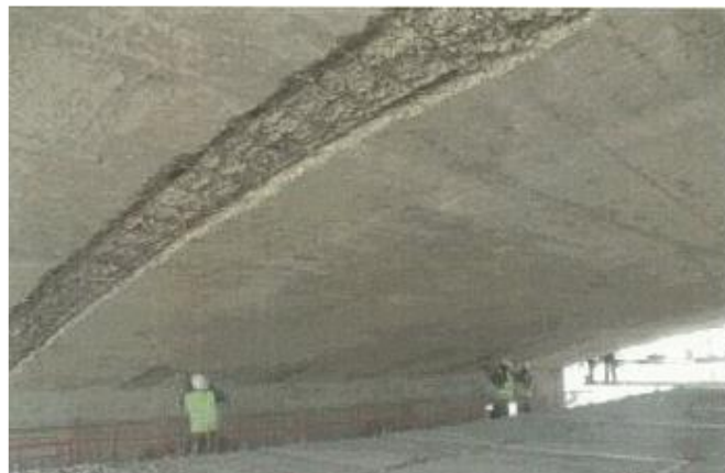
Figure (VIII-3): Damaged concrete removal from ceiling beams
