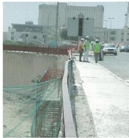
Figure (VIII-83). Removing of old sidewalks on bridge and between them
