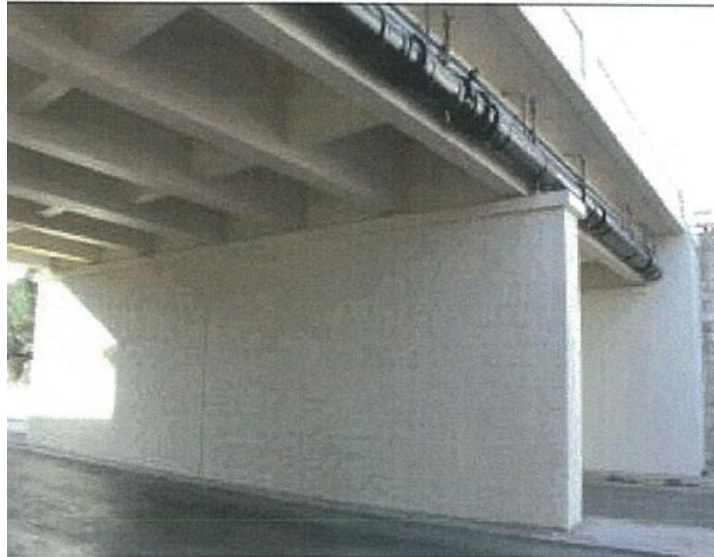
Figure VI-114. AL Sreem Road bridge: view of ceiling and exterior wall
