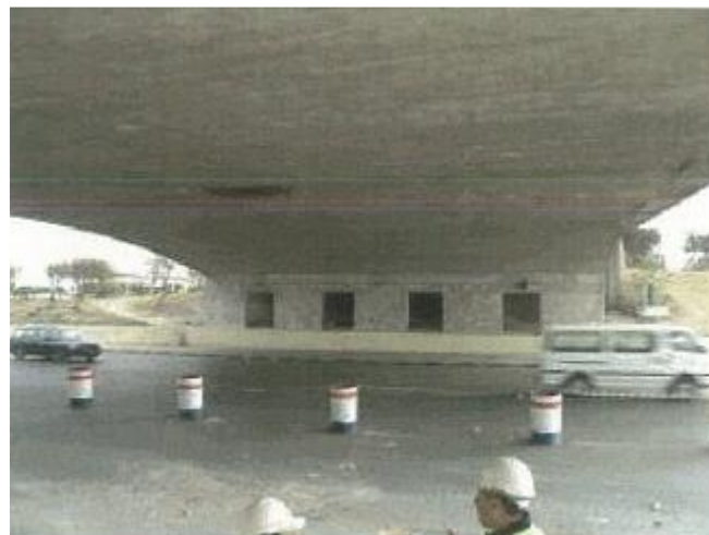
Figure VI-25. View of deck ceiling
