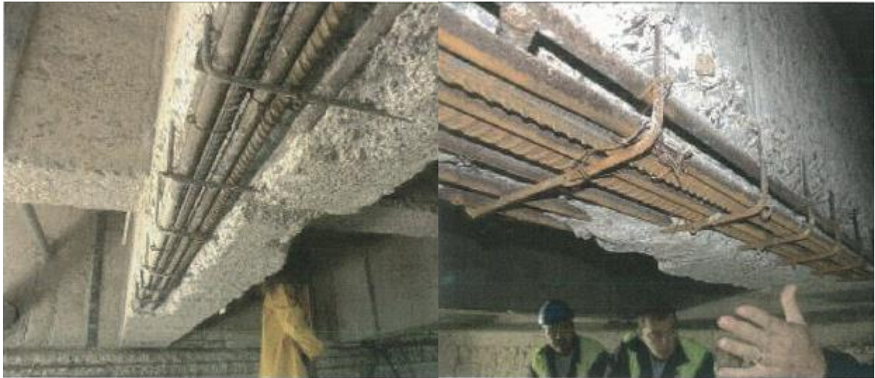
Figure.VIII-144 & VIII-145. Rebar replacement on the damaged longitudinal slab beams
