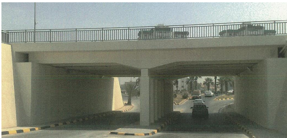
Figure (VIII-190) The view of the concrete bridge elements after application of all recommended measures and materials
