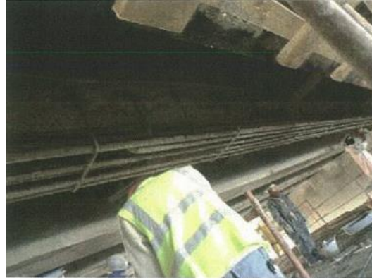
Figure (VIII-163) Reinforcement rods after cleaning, longitudinal slab beam
