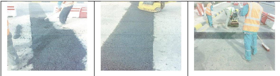
Figure (VIII-195) Placement and compaction of wearing asphalt course
