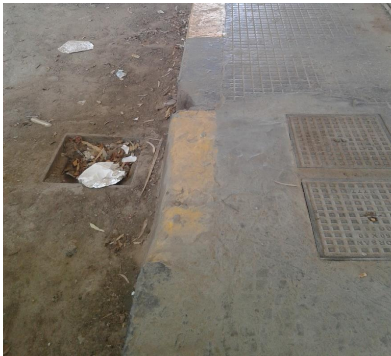
Figure (IX-89) A general view of catch pit under the bridge
