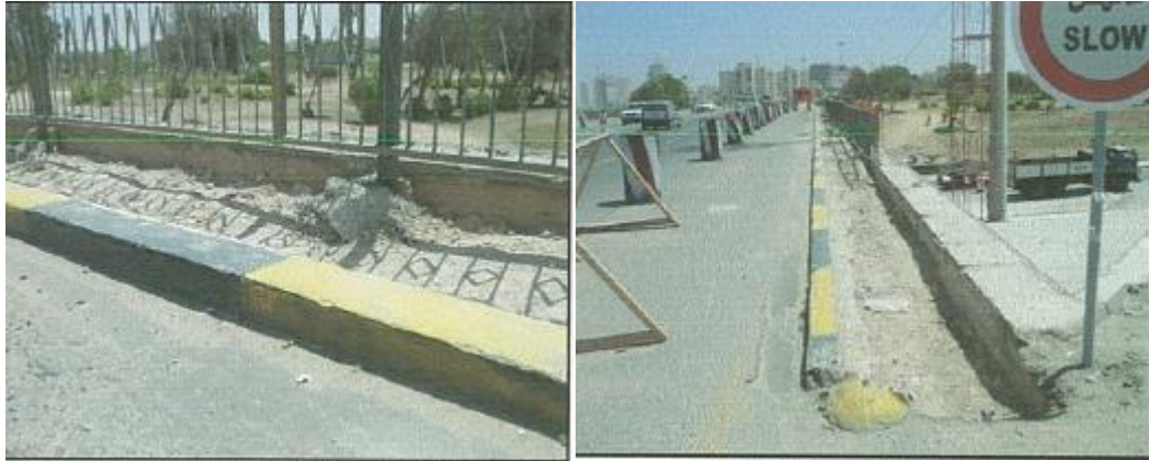
Figure (VIII-21) Removing of old sidewalks on bridge and between them
