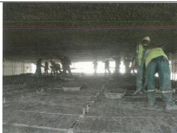
Figure (VIII-111) Finalizing deck ceiling with special mortar
