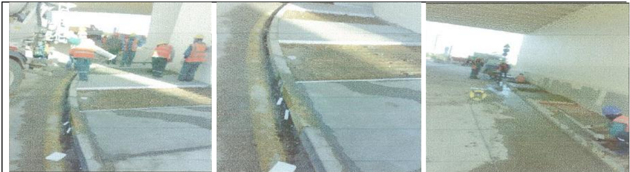
Figure (VIII-172) Execution of a new part of sidewalk under bridge
