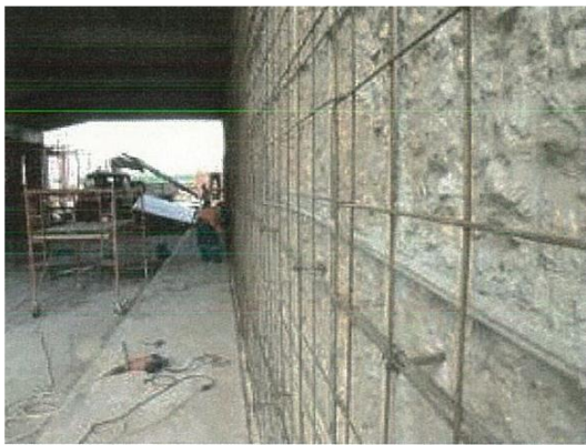
Figure (VIII-188) Repairing of abutment: steel mesh for shrinkage control
