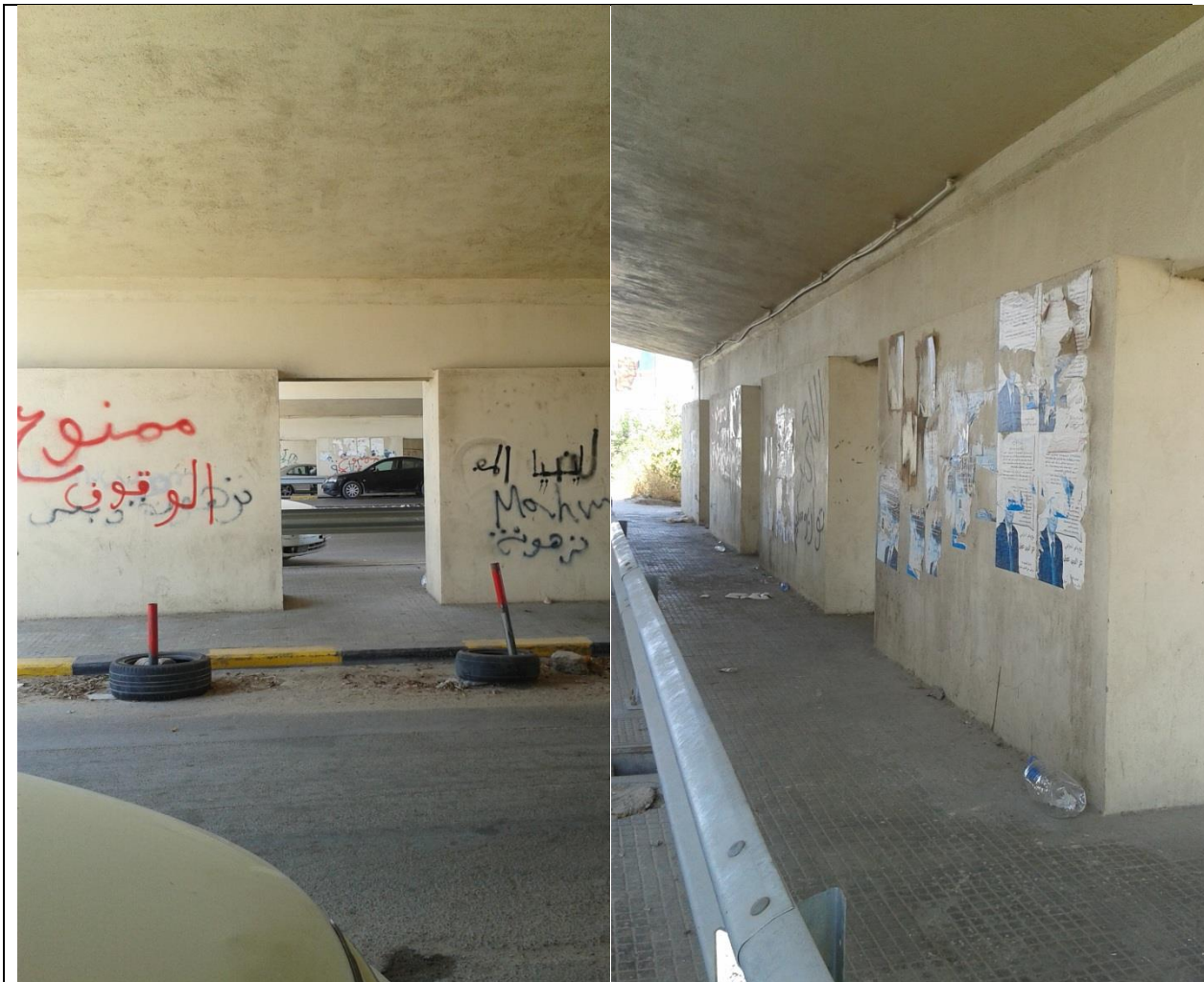
Figure (IX-75) View of supporting wall with ceiling
