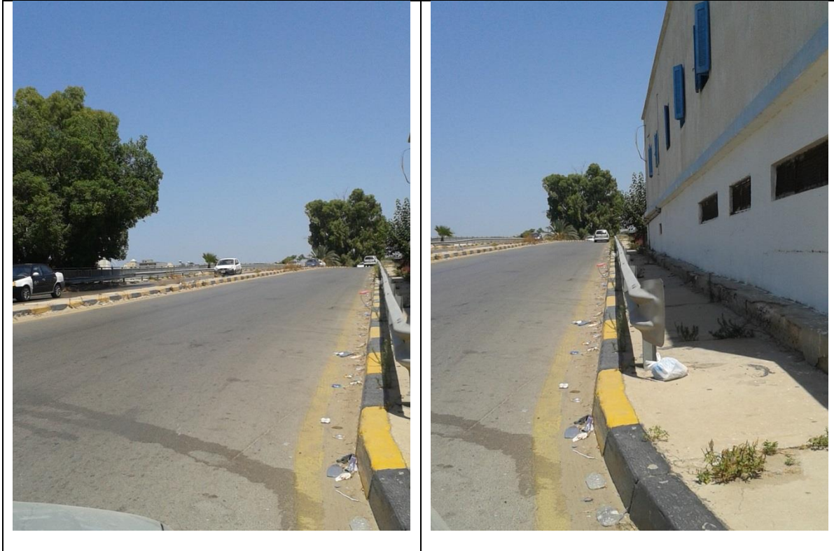
Figure (IX-85) A general view of asphalt wearing layer
