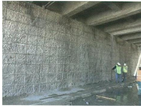
Figure (VIII-187) Reinforcing rebar covered with cementitious protecting material
