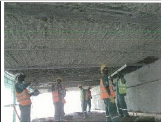
Figure (VIII-107) Finalizing underpass ceiling with cementitious base special mortar
