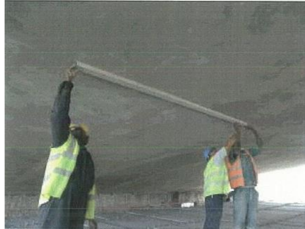
Figure (VIII-66) Deck ceiling slab with special mortar
