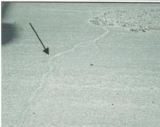
Figure (VIII-92). cracks before injection
