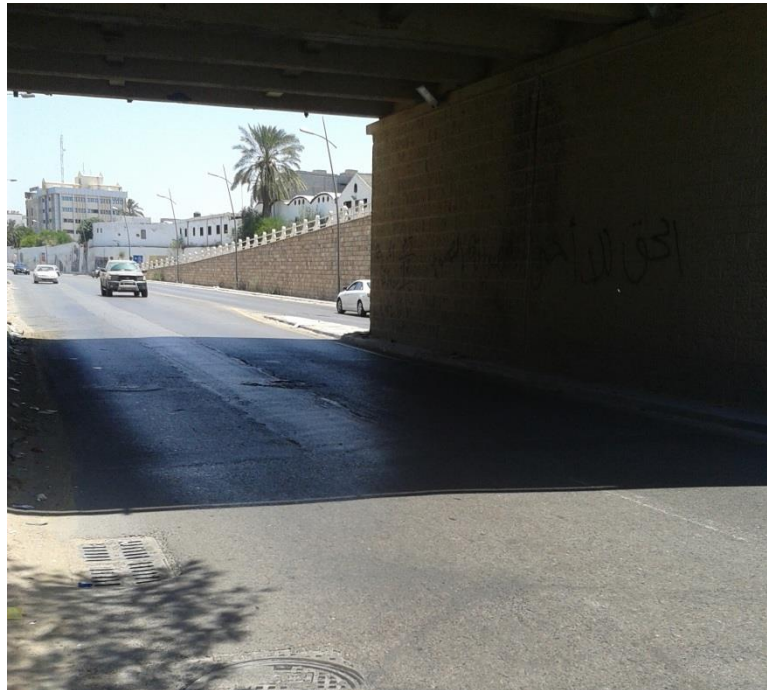
Figure (IX-108) A general view of catch pit under the bridge
