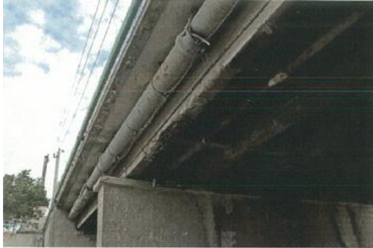
Figure VI-128. View of superstructure of bridge
