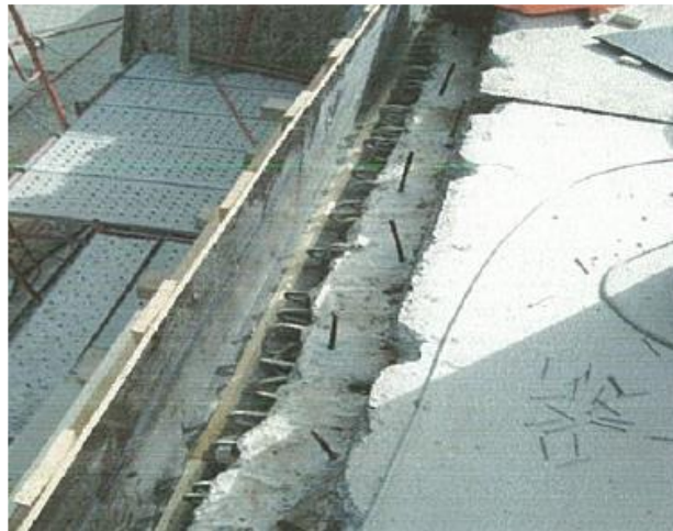
Figure (VIII-104) Removal of old edge beam
