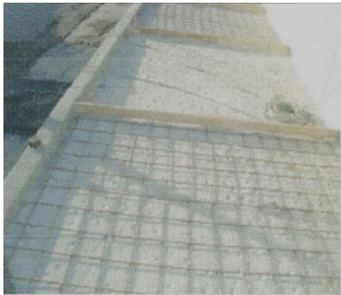
Figure (VIII-152) New wire mesh for new layer of concrete sidewalk
