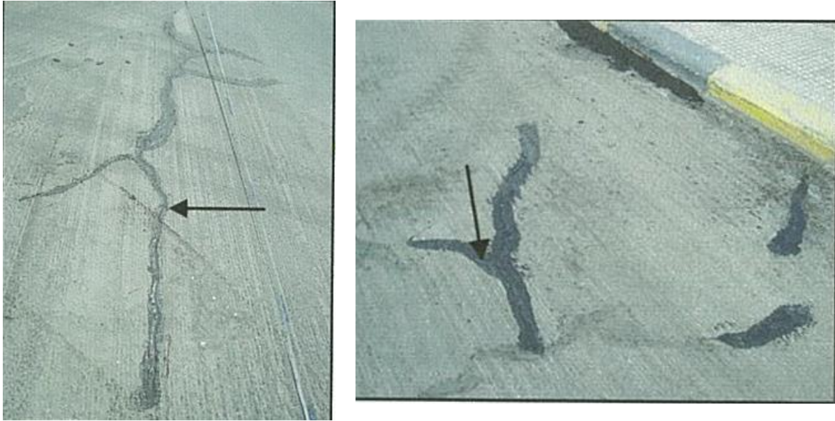
Figure (VIII-93). Cracks after injection
