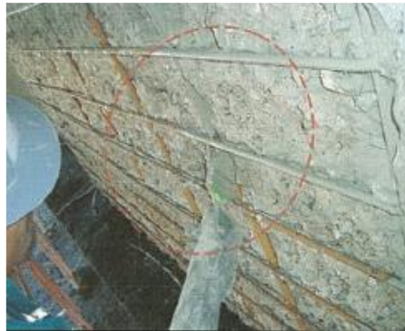
Figure (VIII-12) Application of cementitious base material for protection of rebars
