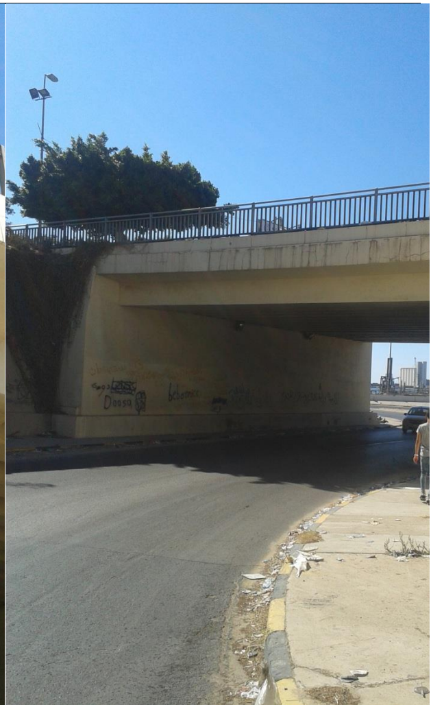
Figure (IX-116) A view of cantilever slabs (south side)
