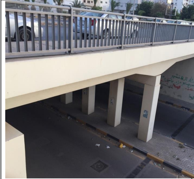
Figure (IX-150) A general view of fences on the bridge
