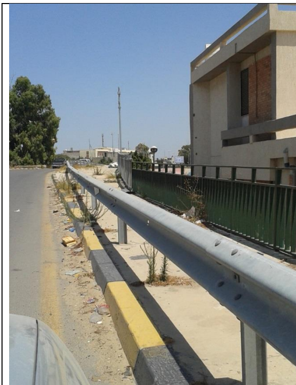
Figure (IX-87) A general view of fences on the bridge
