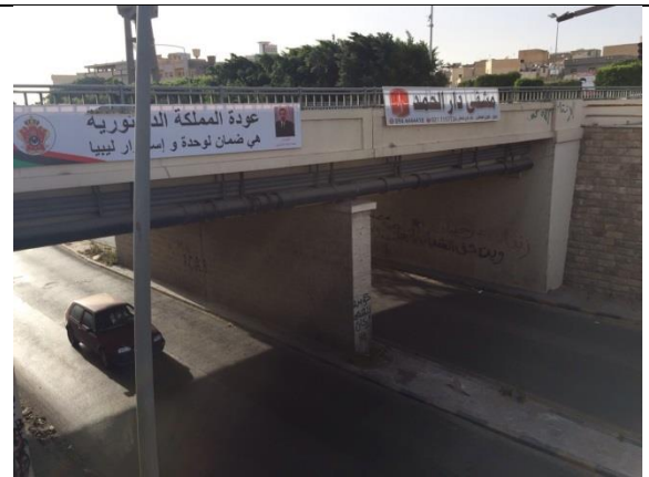
Figure (IX-91) A general view of Al Sreem Road Bridge
