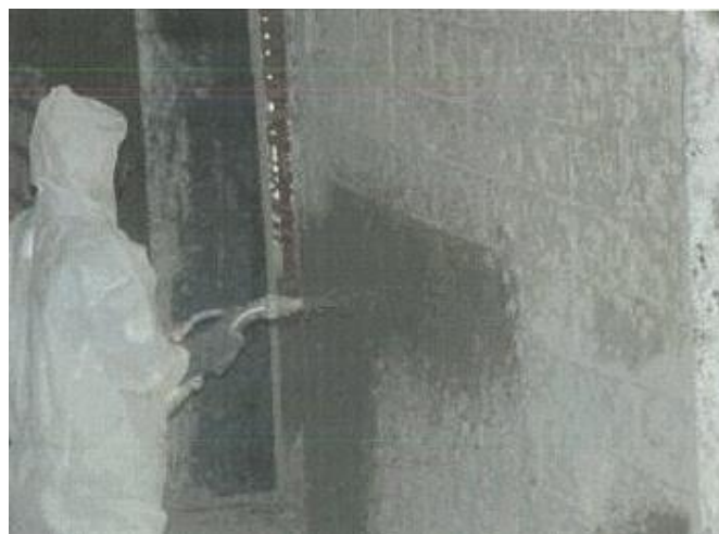
Figure (VIII-17) cementitious base special mortar on exterior walls
