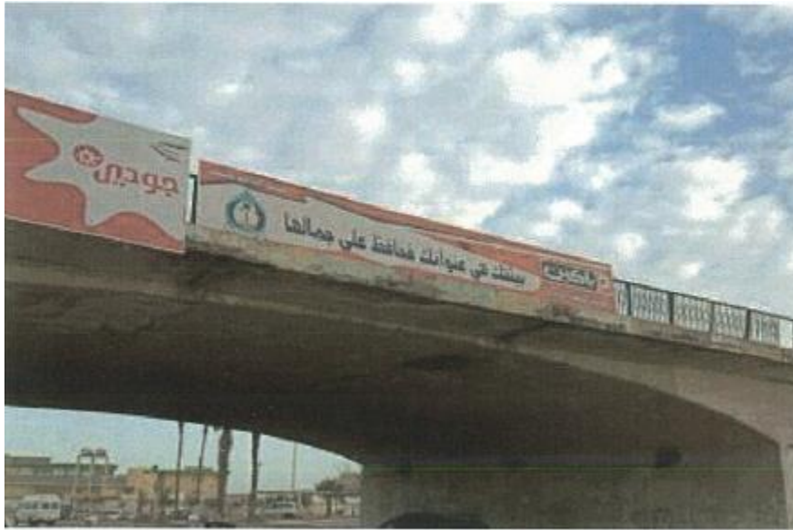
Figure VI-51. General view of the bridge
