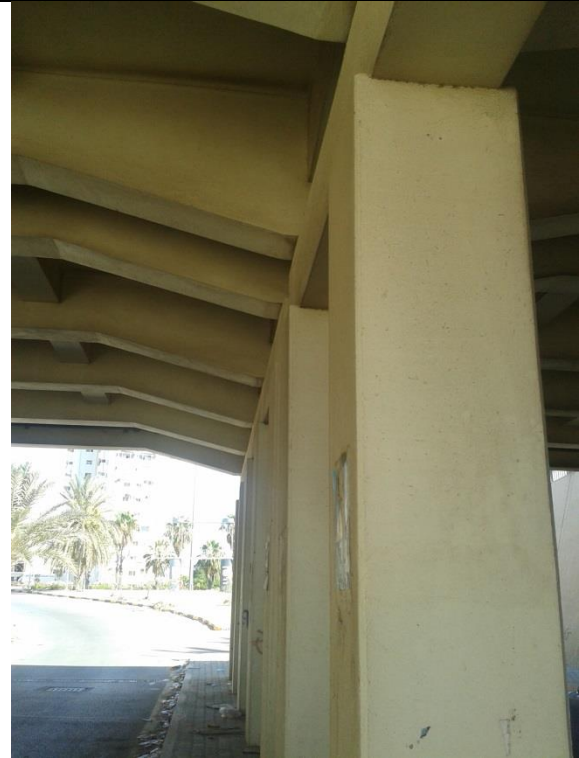
Figure (IX-133) Undamaged concrete surface of strengthened column
