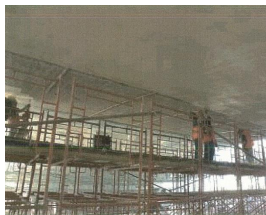
Figure (VIII-79) Finalizing of protecting mortar cover on ceiling
