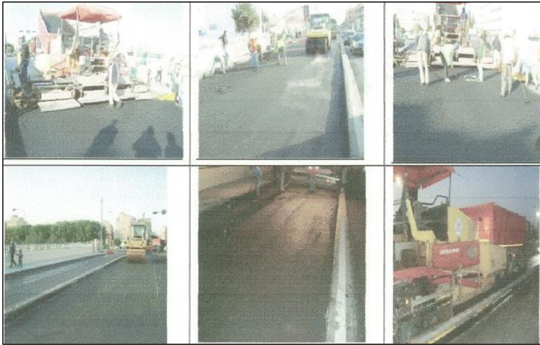
Figure (VIII-156) Placing the new wearing course
