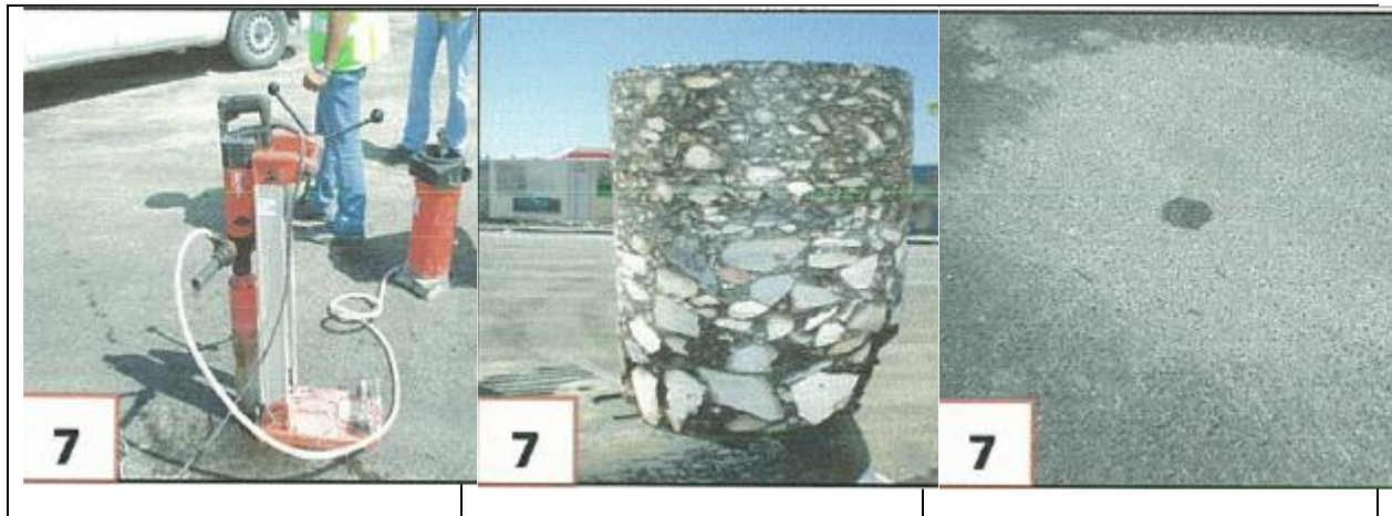
Conti. ....Figure (VIII-44) Phases of placing of bituminous materials
