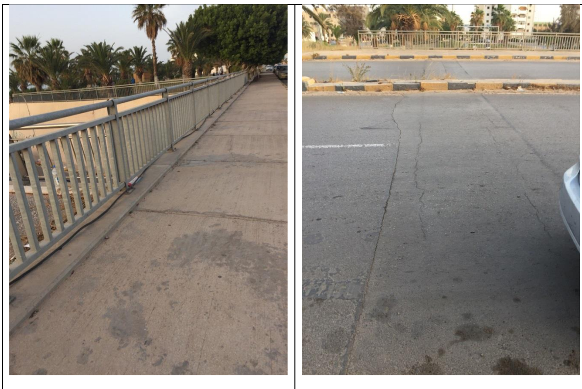
Figure (IX-148) A general view of Pedestrian path on bridge
