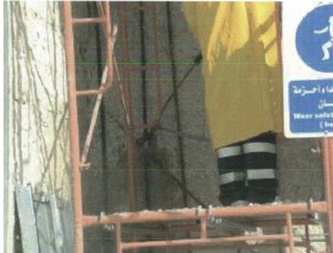
Figure (VIII-9): Rebars cleaning with water-sand blasting on the interior walls
