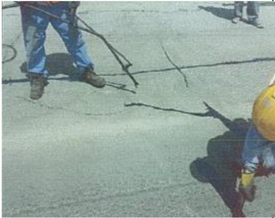
Figure (VIII-42) Injection of cracks by machine
