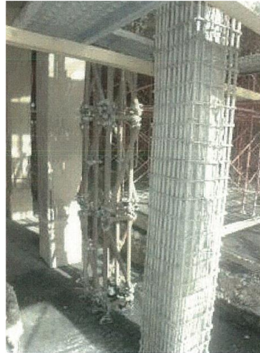
Figure (VIII-183) Column: Protection of rebars with cementitious materials
