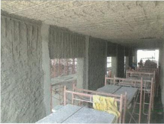
Figure (VIII-67) Cementitious base special mortar on exterior walls
