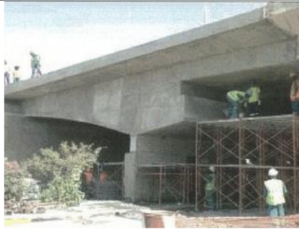
Figure (VIII-110) Finalized lateral beam with special mortar
