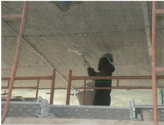
Figure (VIII-76) Rebars protection with cementitious base material
