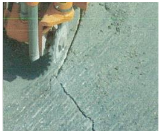
Figure (VIII-40) Opening the crack by special machine
