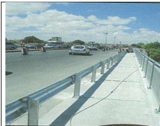
Figure (VIII-55) Fence and guardrail after installation
