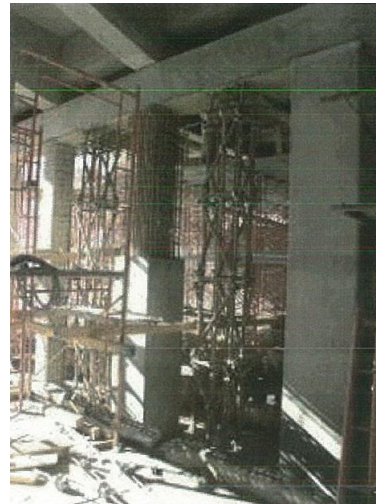
Figure (VIII-183) Column: Protection of rebars with cementitious materials
