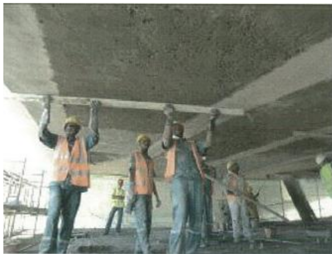
Figure (VIII-16) Deck ceiling slab with special mortar
