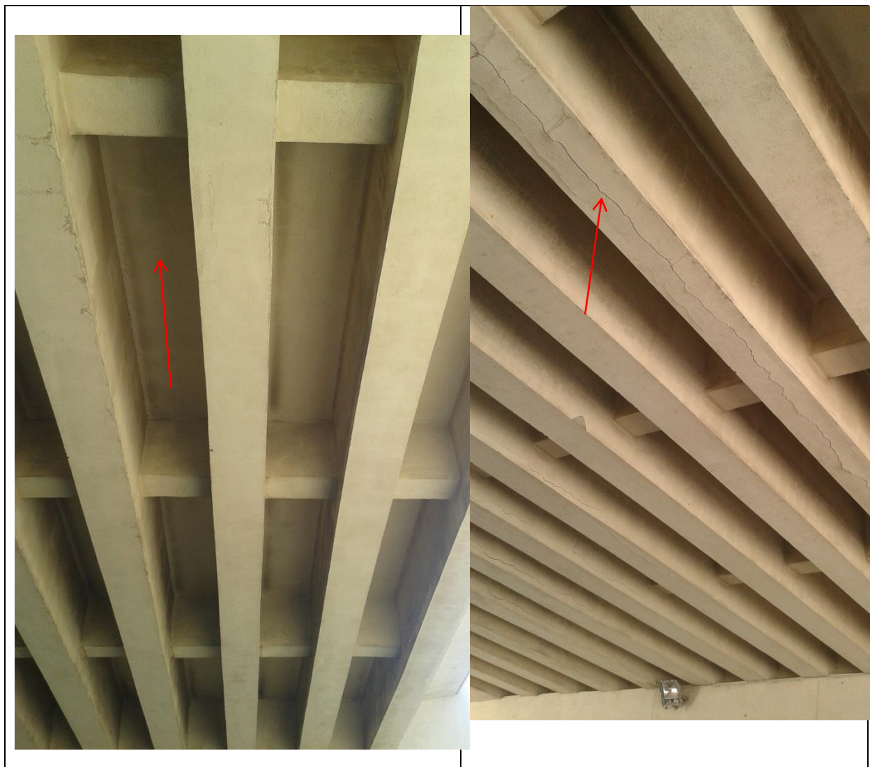
Figure (IX-111) A general view of deck slabs in superstructure of bridge
