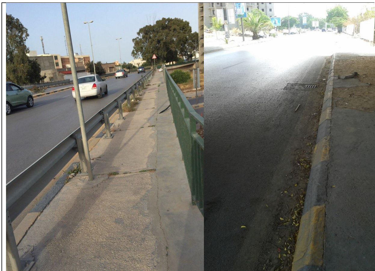
Figure (IX-57) A general view of Pedestrian path on bridge
