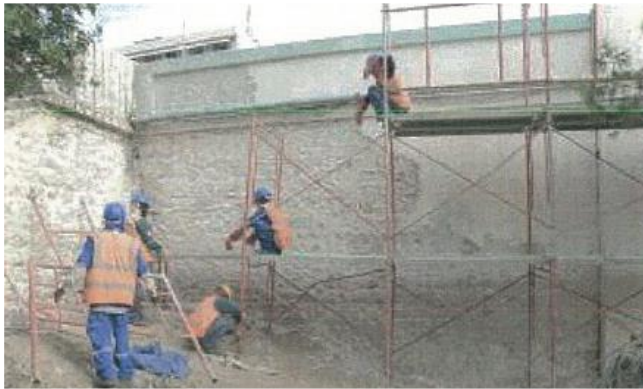
Figure (VIII-141) Damaged plastering and concrete removal from the abutments and sidewalk
