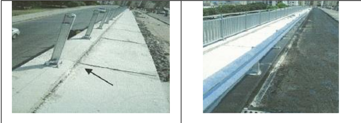
Figure (VIII-31) Columns for fences over beam and fence and guard rail after assemblage
