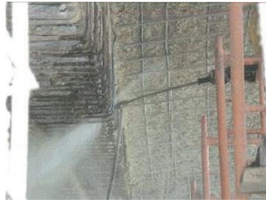
Figure (VIII-62) Rebars cleaning with water-sand blasting on lateral beam
