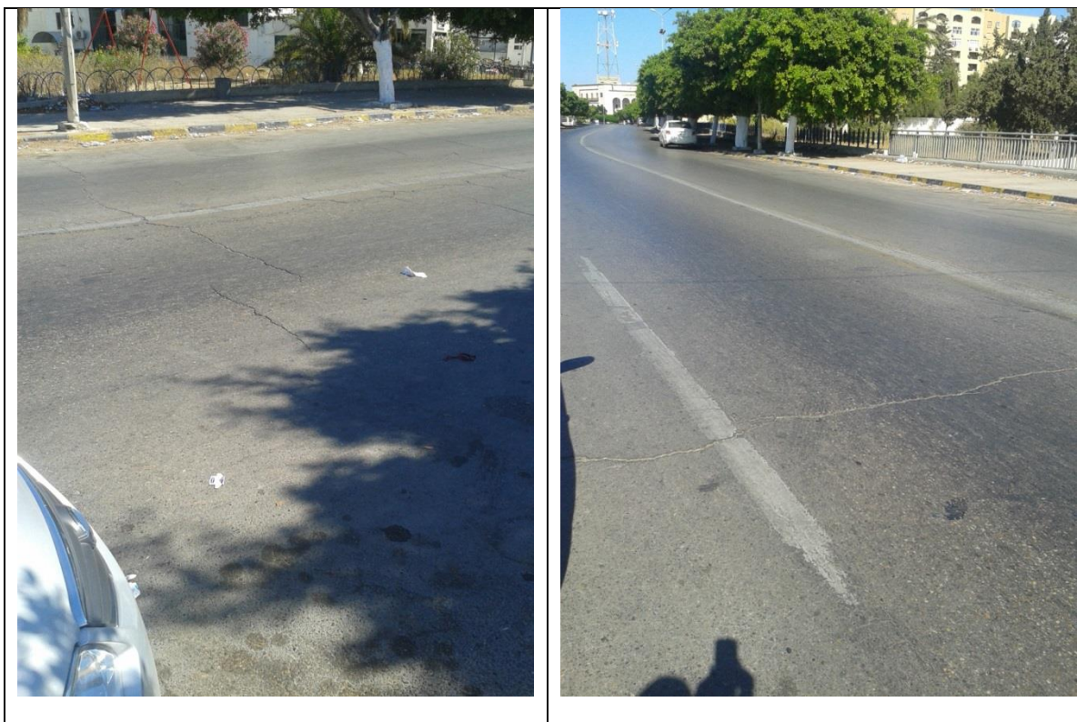
Figure (IX-123) A general view of asphalt wearing layer
