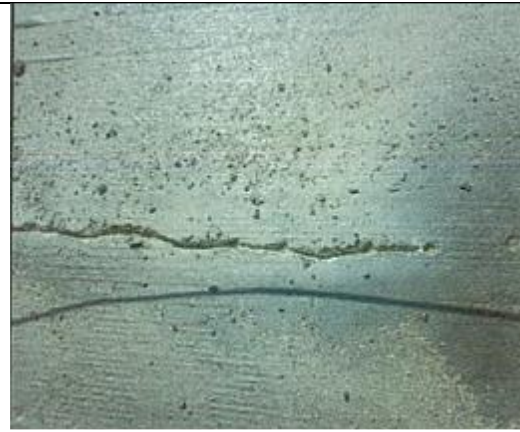
Figure (VIII-40) Opening the crack by special machine
