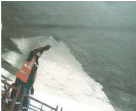
Figure (VIII-69) Application of protecting coating on ceiling by roller
