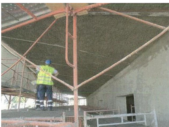
Figure (VIII-78) Execution of new protecting mortar cover on ceiling
