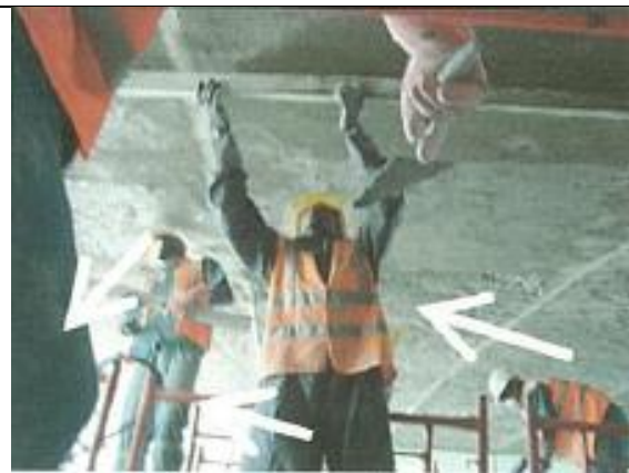
Figure (VIII-112) plastering for ceiling
