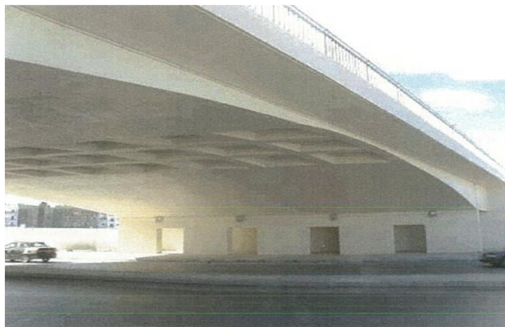
Figure VI-60. Alsseka bridge ceiling and cantilever
