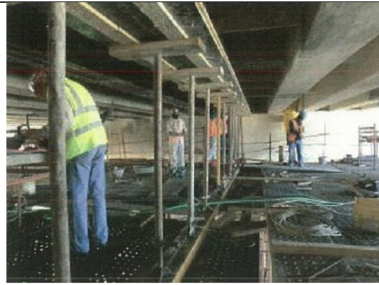
Figure (VIII-165) Longitudinal slab beam bottom grouting
