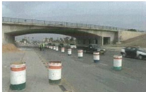
Figure VI-2. Souk Athulatha1 Bridge, south side
