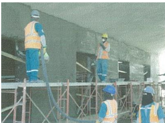
Figure (VIII-80) Plastering of exterior wall
