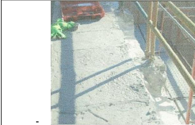
Figure (VIII-170) Removal of "old" beam for fence
