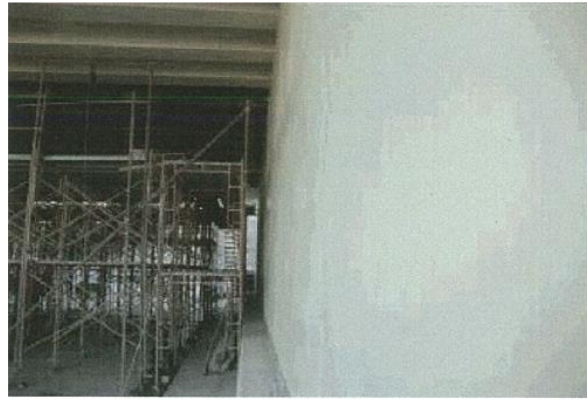
Figure (VIII-169) View of abutment wall after plastering and painting
