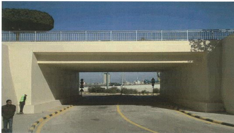
Figure VI-132. View of Alshaab Port Bridge
