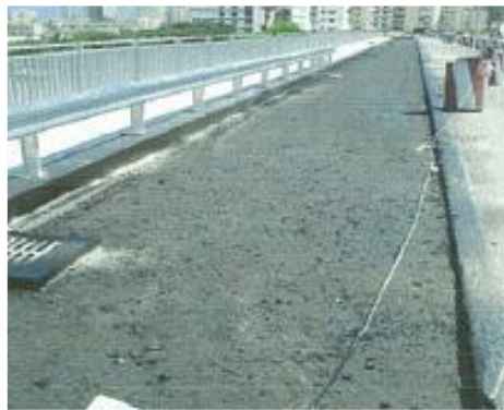
Figure (VIII-48) Sub base after spray MC
