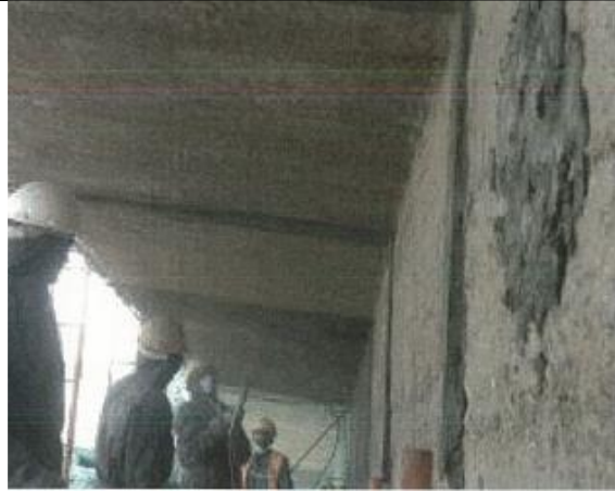
Figure (VIII-109) Finalizing cantilevers and lateral beam with special mortar
