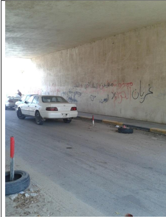
Figure (IX-79): General view of abutment
