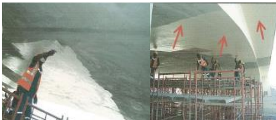
Figure (VIII-19) Application of protecting coating on ceiling by roller
