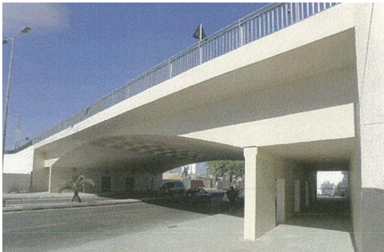
Figure (VIII-100) Al Seeka Bridge after all repair measures.
