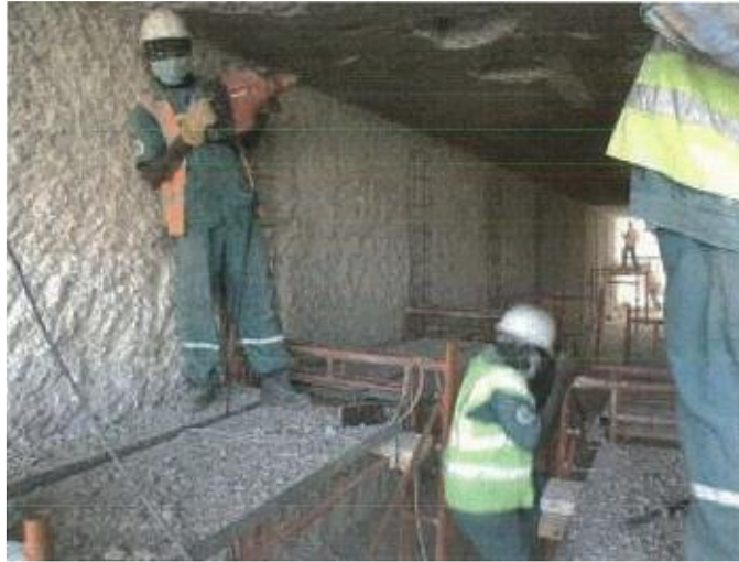
Figure (VIII-60) Damaged concrete removal from tunnel ceiling
