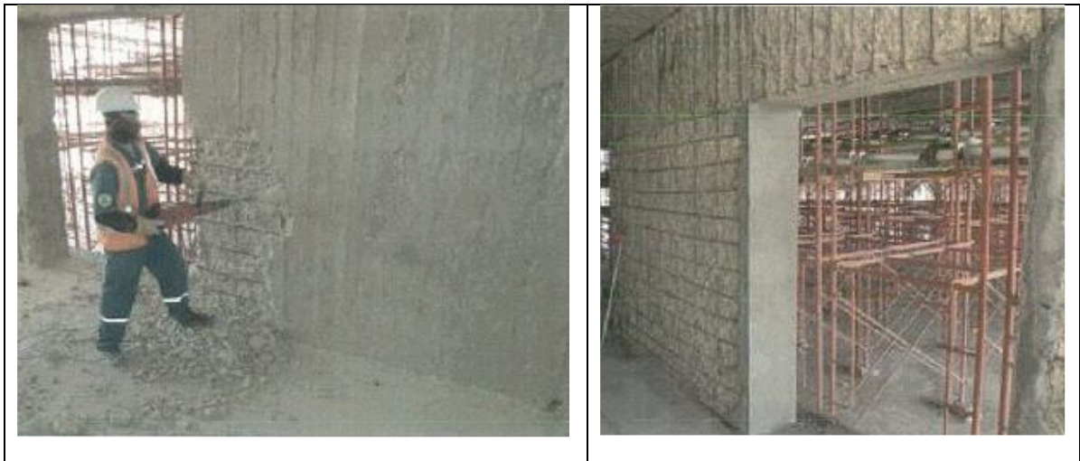
Figure (VIII-2) Damaged concrete removal from exterior walls
