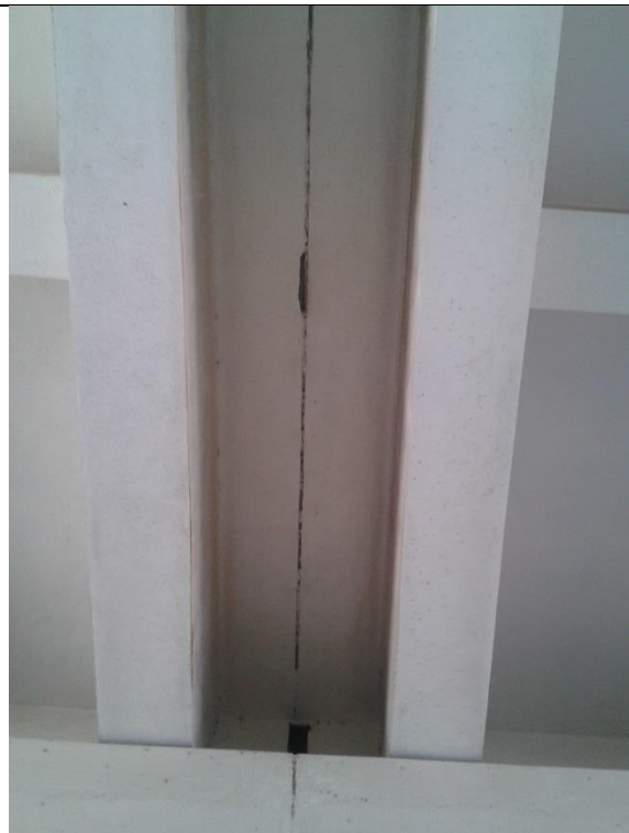
Figure (IX-147) View of characteristic part of expansion joints
