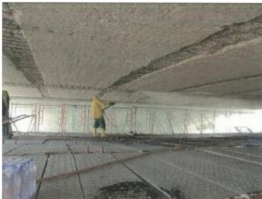
Figure (VIII-61) Rebars cleaning with water-sand blasting in deck ceiling slab
