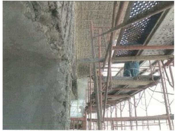
Figure (VIII-64) Rebars protective coating on cantilever
