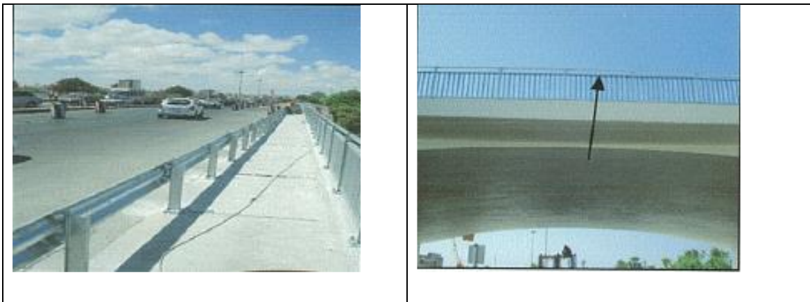
Figure (VIII-32) fence and guard rail after assemblage
