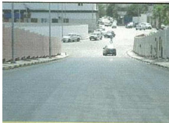
Figure (VIII-95). The road after finish asphaltting
