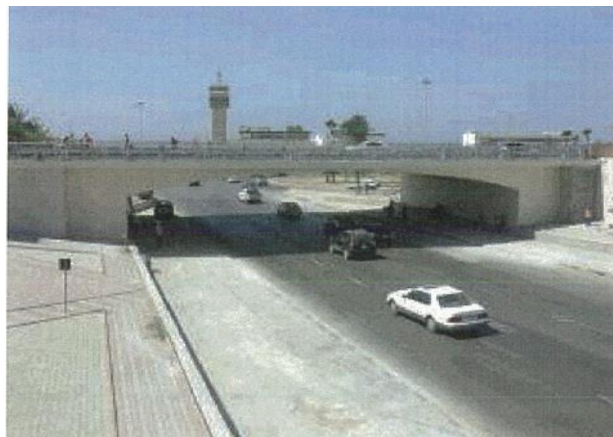
Figure VI-29. Souk Athulatha 2 bridge, south side
