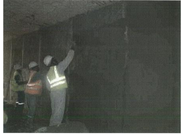
Figure (VIII-68) Levelling on the interior walls
