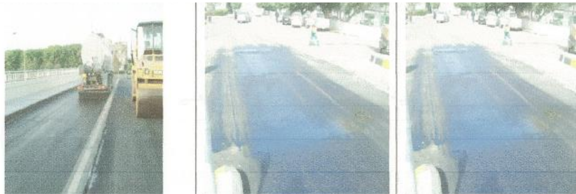
Figure (VIII-155) Spreading tack coat (RC2)
