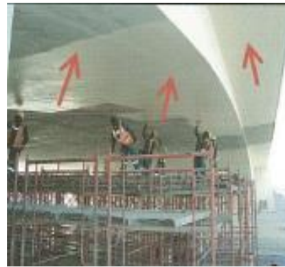
Figure (VIII-69) Application of protecting coating on ceiling by roller
