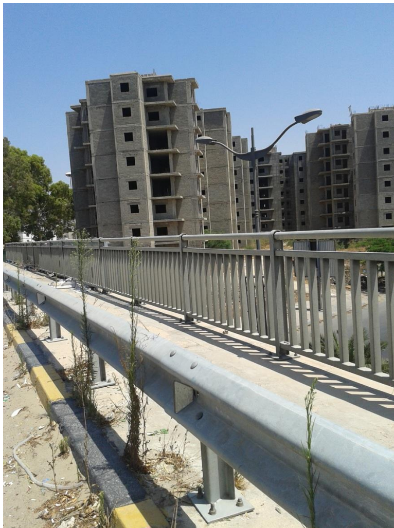
Figure (IX-63) A general view of guardrail on the bridge
