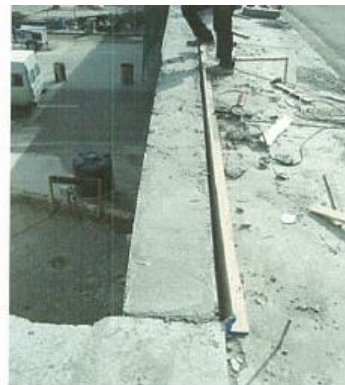
Figure (VIII-29) Casted edge beam
