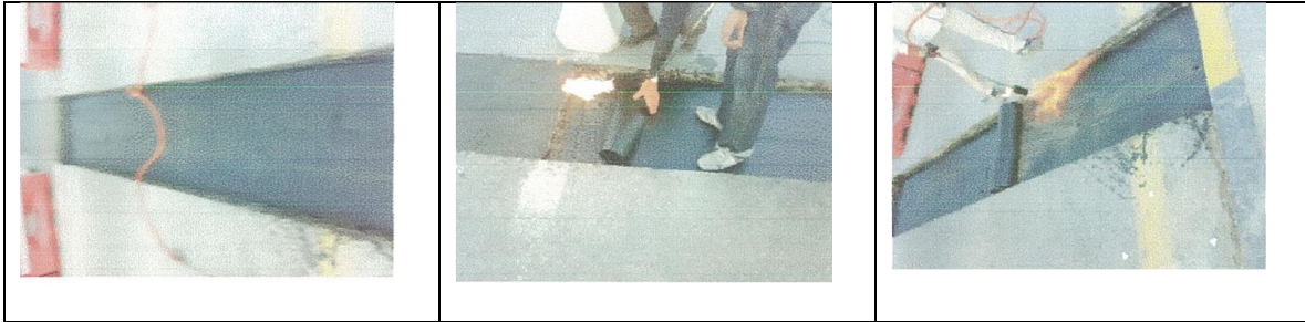
Figure (VIII-194) fixing of water proofing membrane
