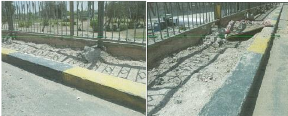
Figure (VIII-6): Sidewalk on bridge
