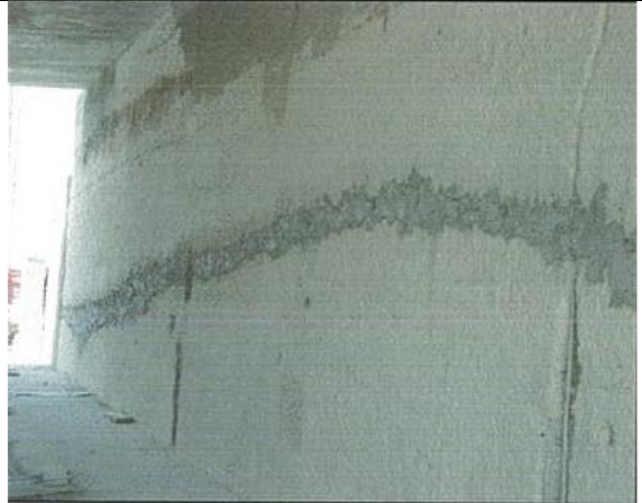
Figure (VIII-114) The crack in abutment prepared for injection
