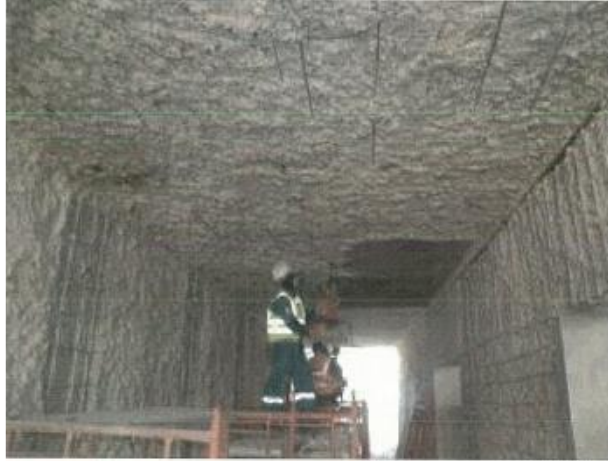
Figure (VIII-4): Damaged concrete removal from tunnel ceiling
