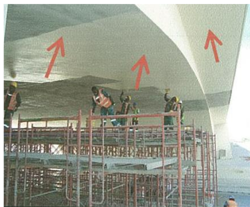
Figure (VIII-81) Painting of repaired surfaces of bridge elements
