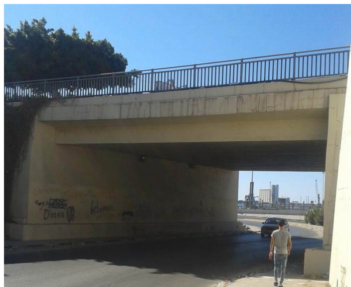
Figure (IX-110) A general view of Al shaab port bridge
