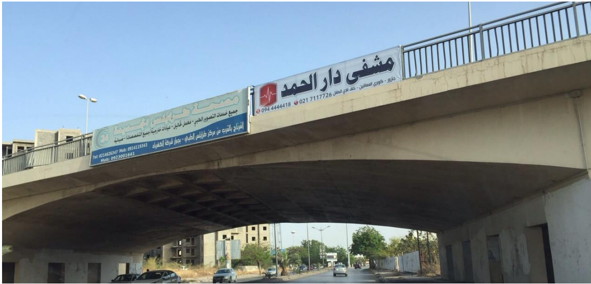
Figure (IX-45) A View of Lateral beams
