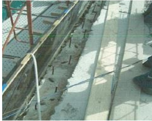
Figure VIII-1. Removal of "old" edge beam
