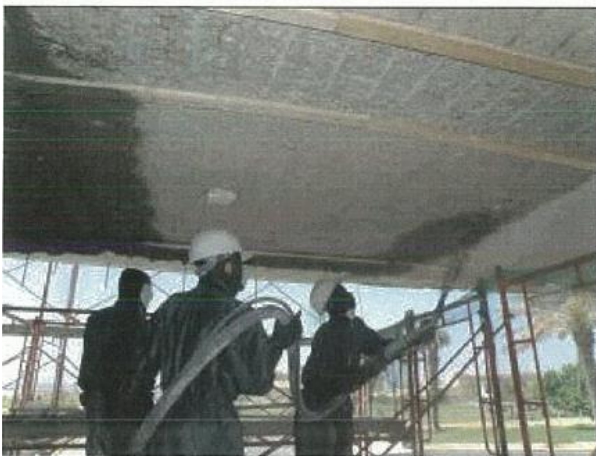
Figure (VIII-65) Cementitious base special mortar on deck ceiling beams
