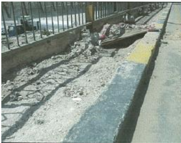
Figure (VIII-83). Removing of old sidewalks on bridge and between them
