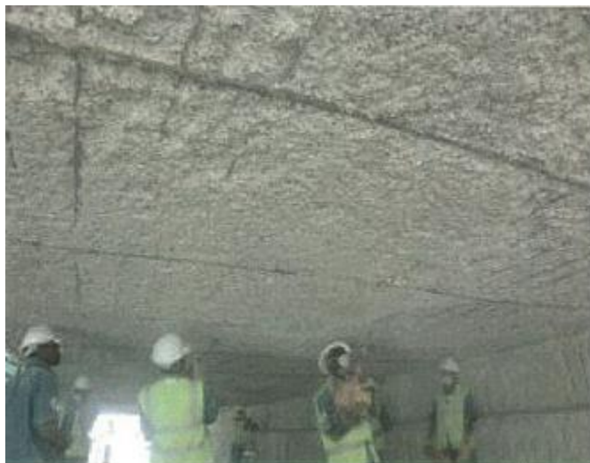
Figure (VIII-101) Damaged concrete removal from deck ceiling slab
