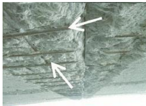
Figure (VIII-10): The view of reinforcement rods after cleaning by mixed water- sand blasting method
