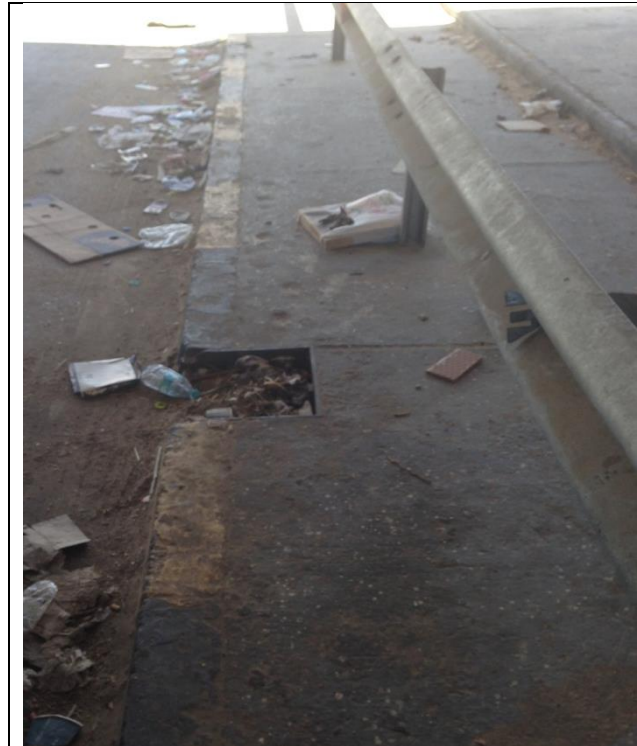
Figure (IX-22) A general view of catch pit under the bridge
