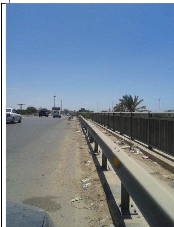
Figure (IX-39): A general view of fences on the bridge
