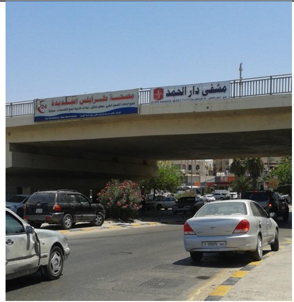
Figure (IX-66) A general view of Bab Bin Gheshir road bridge, middle part
