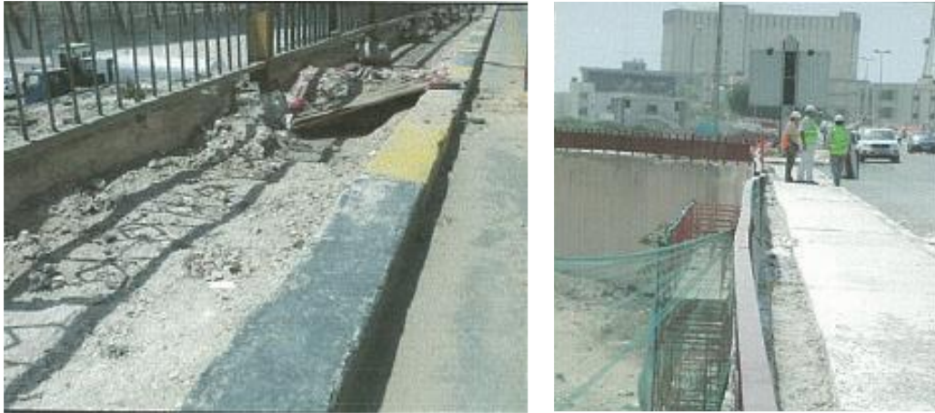
Figure (VIII-120) Removing of old sidewalks on bridge and between them
