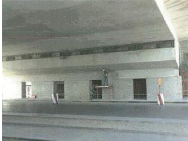
Figure VI-108. View of deck ceiling and exterior wall
