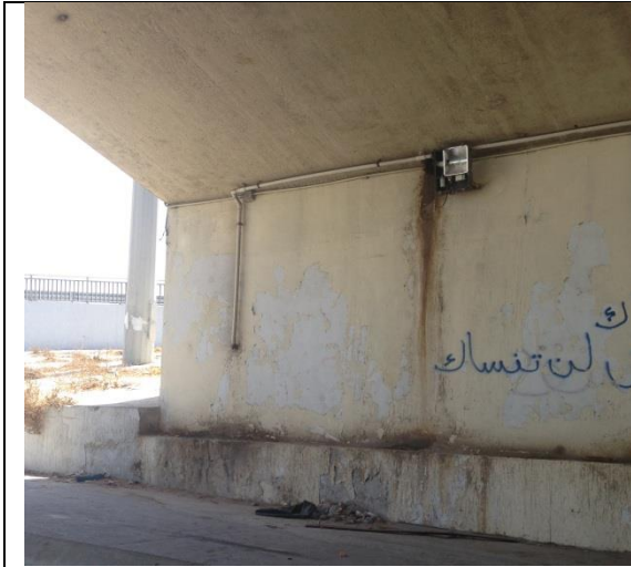
Figure (IX-12) View of supporting wall
