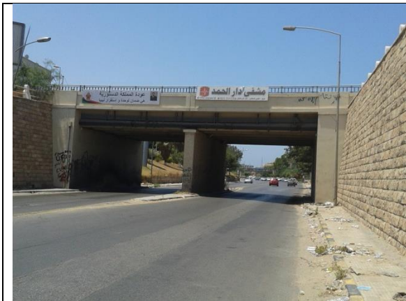
Figure (IX-90) A general view of Al Sreem Road Bridge
