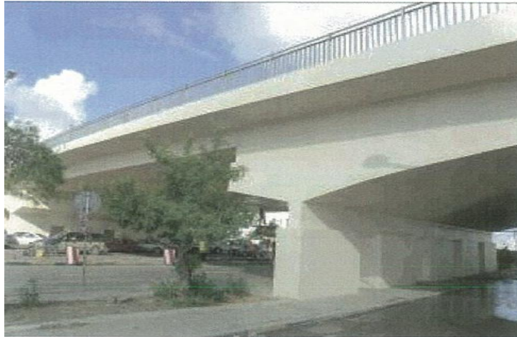
Figure VI-90. Bab Bin Ghashir road bridge view
