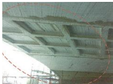
Figure (VIII-75) Local removal work on ceiling of simple beam
