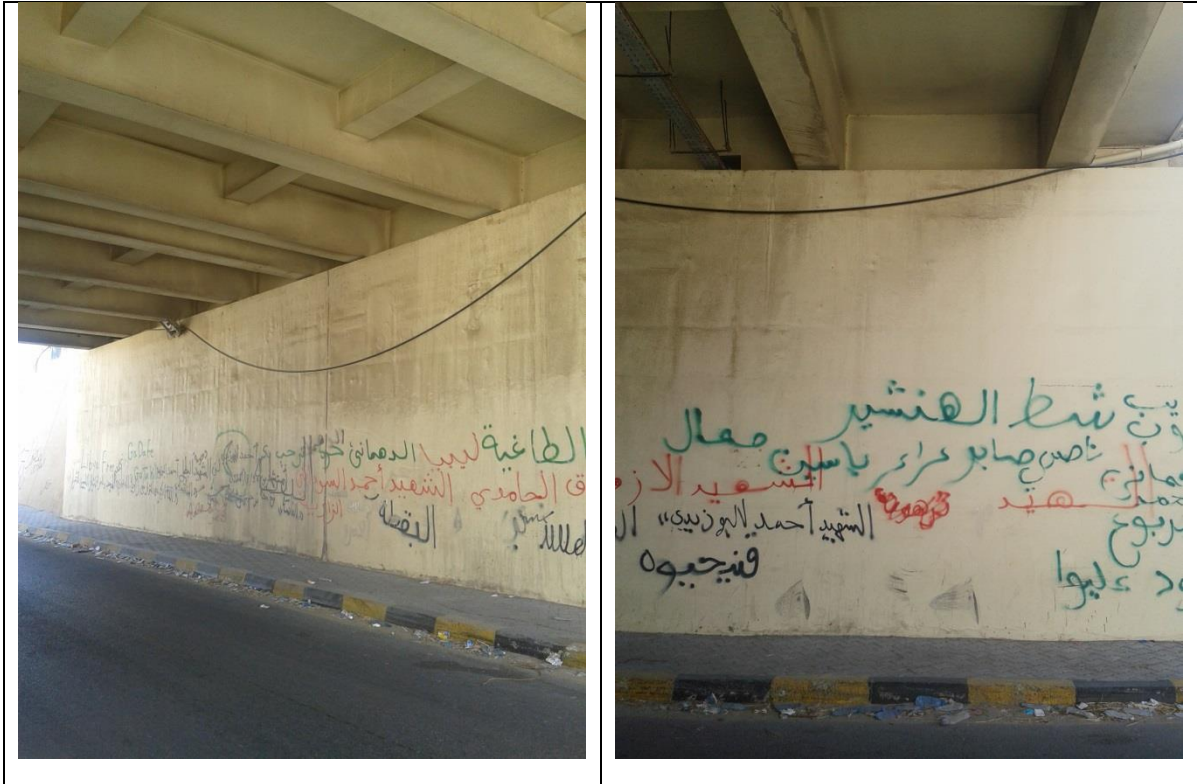
Figure (IX-136) View of strengthened abutment
