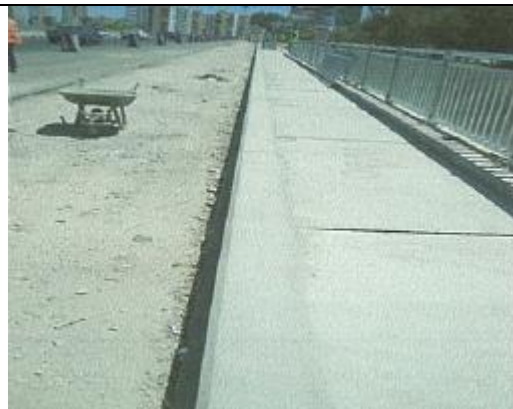
Figure (VIII-30) New side walk on area between two bridges and new curb stone
