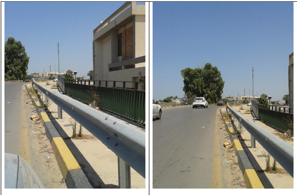
Figure (IX-83) A general view of Pedestrian path on bridge
