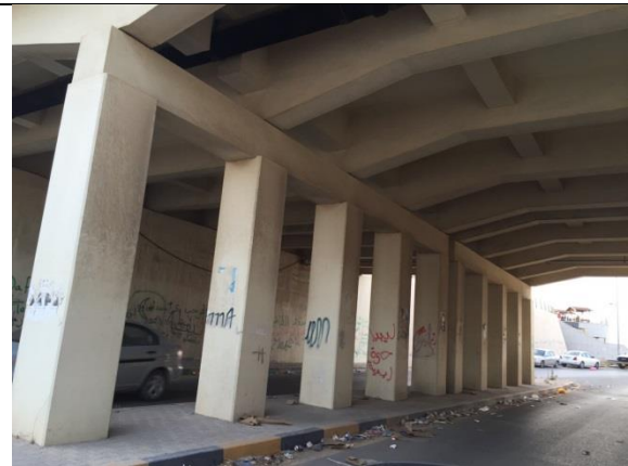
Figure (IX-135) A View of strengthened columns
