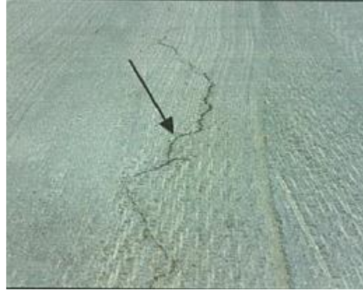
Figure (VIII-92). cracks before injection
