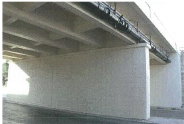
Figure (VIII-151) View of bridge after repairing and painting measures
