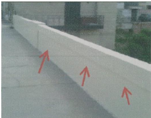
Figure (VIII-150) Repaired and painted concrete part of fence
