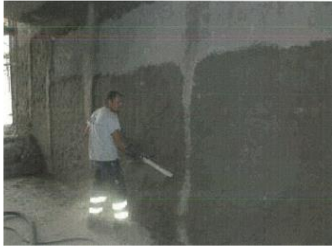
Figure (VIII-18) Levelling on the interior walls
