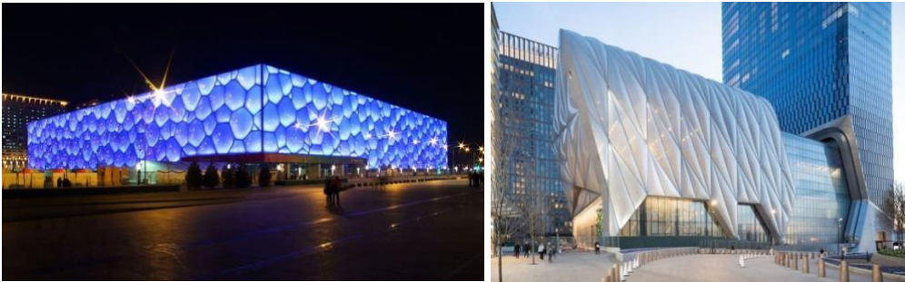
Slika 21(levo) - The Water Cube-Nacionalni plivački centar uPeking, ETFE tkanina (Izvor: Craig Long, A., Design and manufacture of textile composites, Manchester, England Textile Institute, 2007.)
