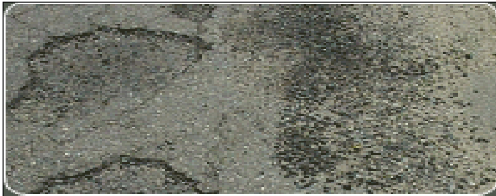
Figure 3.3 Raveling distress in Libyan roads characteristic
