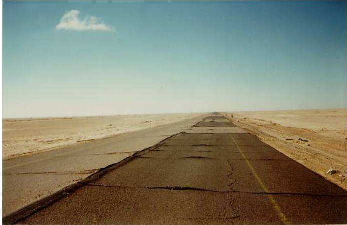
Figure 2.2 The effects of temperature and solar radiation on pavement
