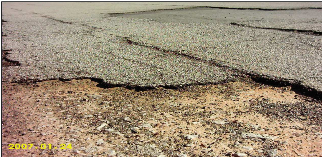
Figure 3.8 Edge damages in Libya roads
