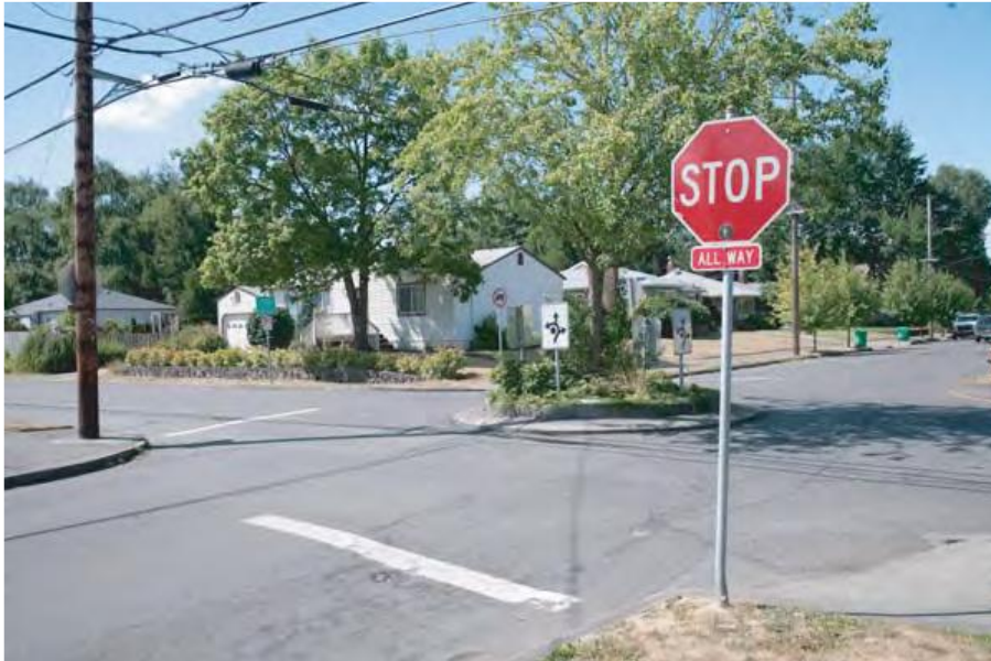
Slika 2.13. Kružna raskrsnica sekundarne putne mreže, Portland, Oregon (SAD) *Izvor: NCHRP Report 672: Roundabouts: An Informational Guide (2010), Exhibit 1-5.
