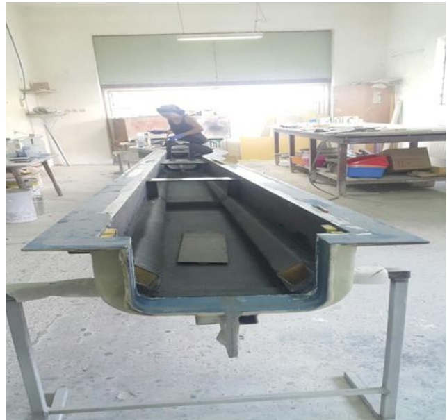
Figure 6.4: Fixing of the stringers and vertical rib on the structure
