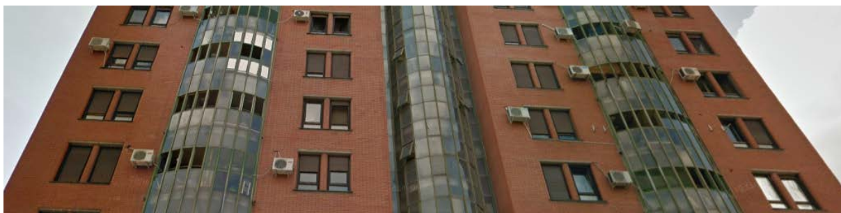
Sl. 4.43 – Detalji fasade stambene kule BCL-5: fugovana opeka
