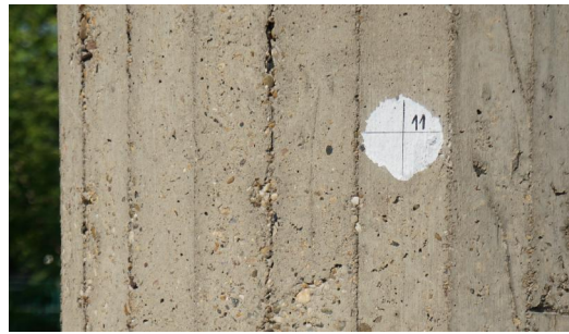
Figure 4.3. Marker point with precisely measured coordinates placed on a concrete column.
