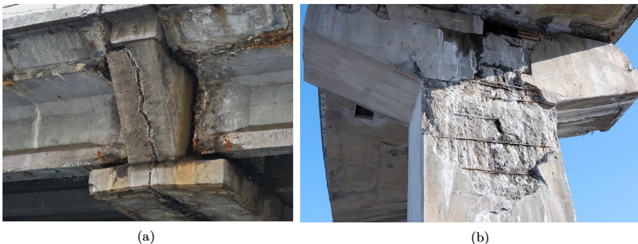
Figure 2.6. Damaged piers: (a) Cracked pier cap, (b) large spalling on the pier.
