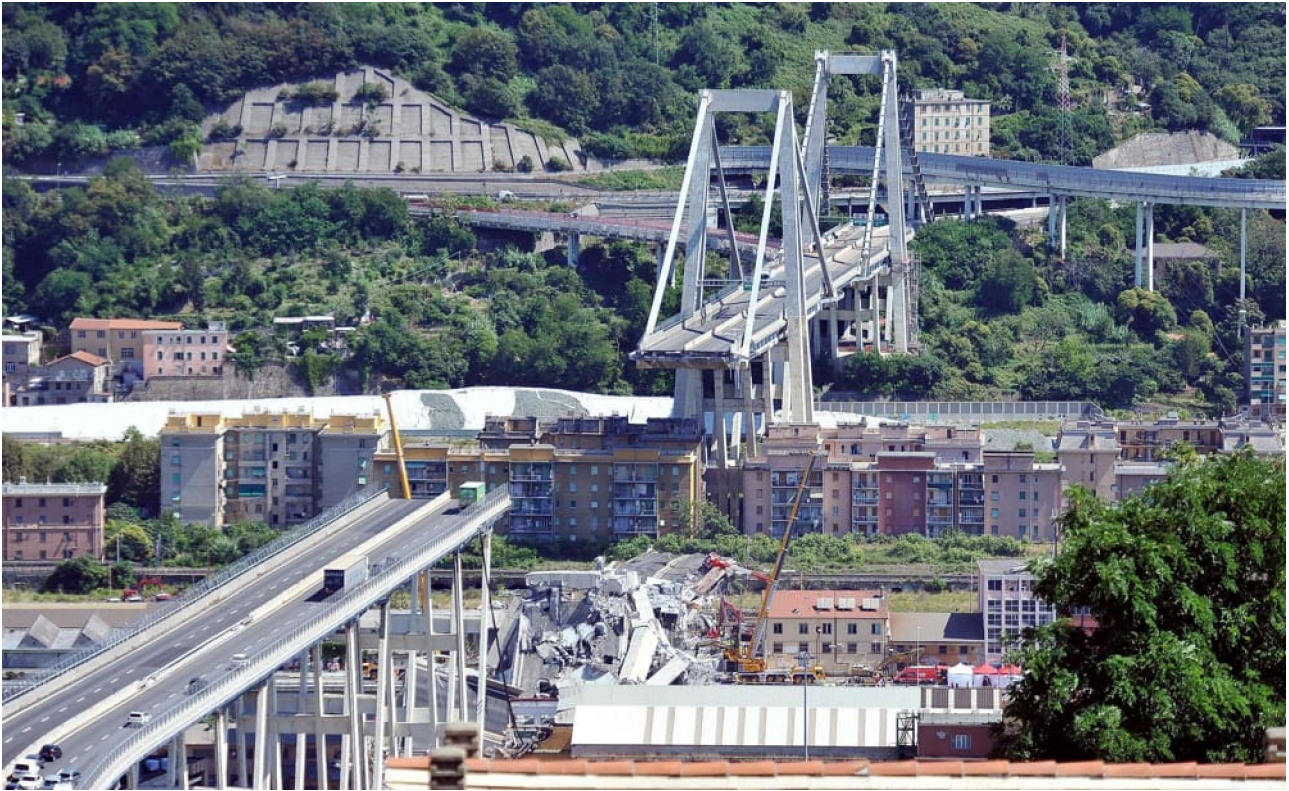
Figure 1.1: Collapse of Morandi bridge in Genoa, on August 14 th 2018 (retrieved from [9])
