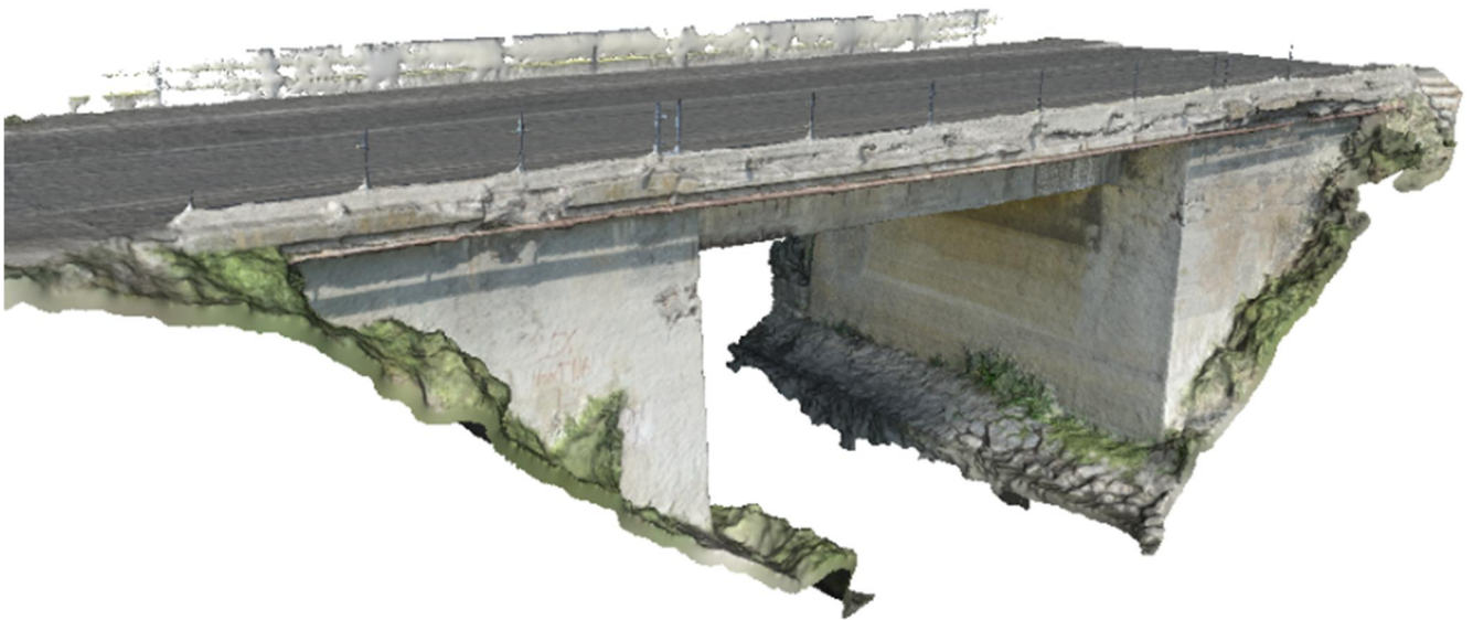
Figure 5.7. The result of 3D Scene Reconstruction: triangulated mesh with texture.
